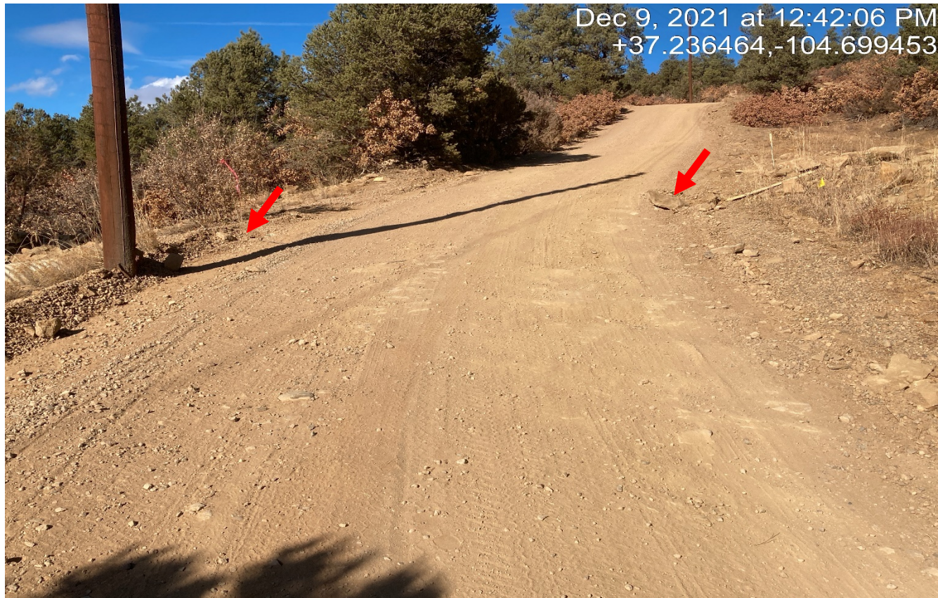
Photo 2. The access road has been regraded however there are steep areas with insufficient gravel and stabilization. The red arrow points to a culvert that was damaged from grading. Lat/Long:37.23640,-104.69944. There is also a rock puled up on the road.
