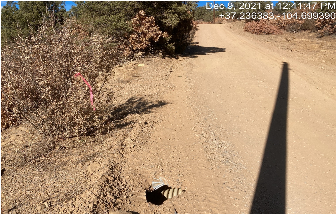
Photo 3. The culvert was damaged which can puncture a tire. This needs to be repaired. There is sand and gravel filling into the opening of the culvert.
