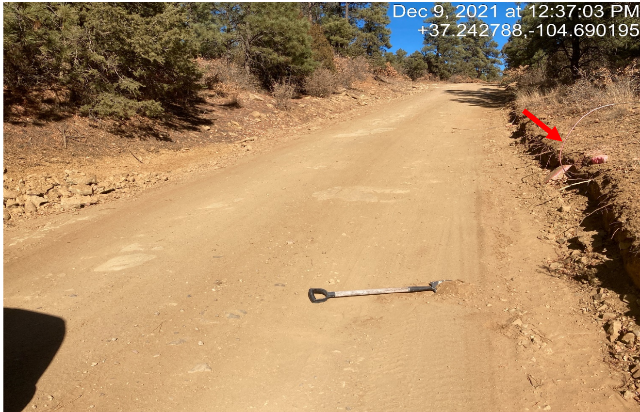
Photo 4. This steep area of the road was regraded however there is now loose soils shown by shovel. This area needs to be stabilized (e.g. gravel, road base). There is also an exposed wire at red arrow.
