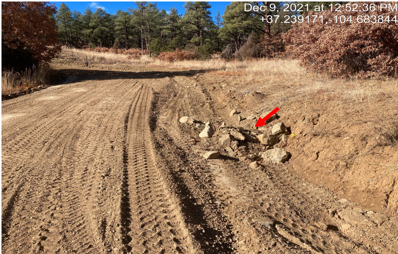
Photo 3. The rock check dam at red arrow is not properly installed. There is loose gravel that needs to be compacted.
