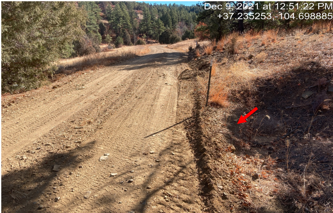
Photo 1. Facing southeast along the access road. The culvert along the road is filled in with sediment. Previous corrective action was not performed.
