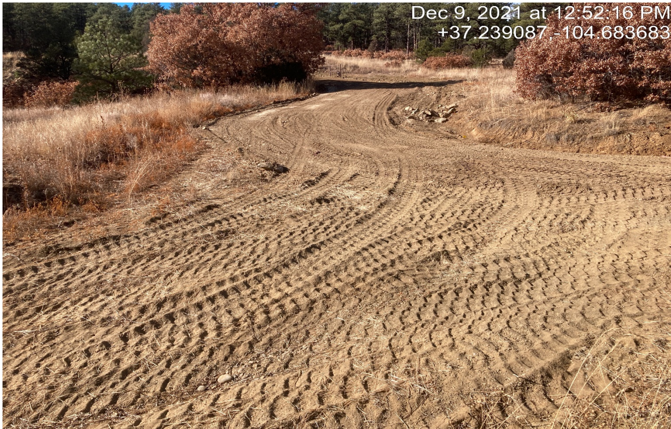
Photo 2. Facing west toward the access road near the location. The road was graded where vehicle rutting has occurred. There is disturbance shown in the bottom left of the photo that needs to be seeded and reclaimed.
