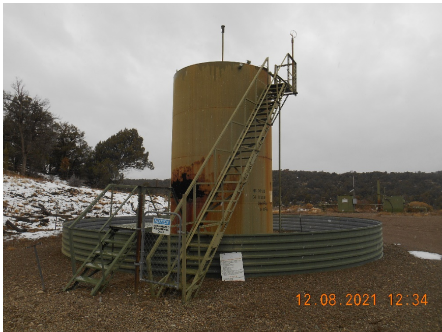
Tank battery. Rusted out.
