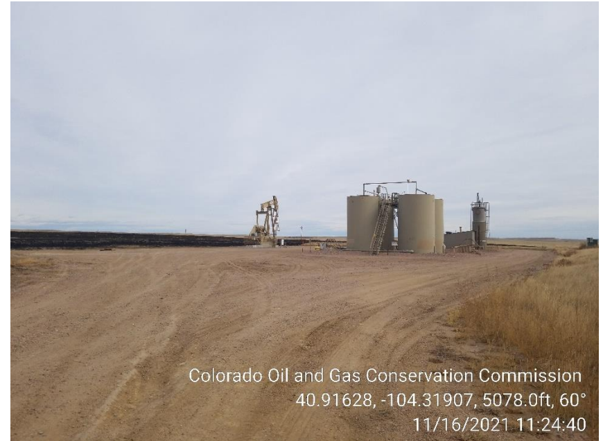
Photo 2 – Tank Battery
