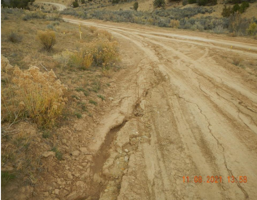
Access road surface and ditch are storm water damaged.
