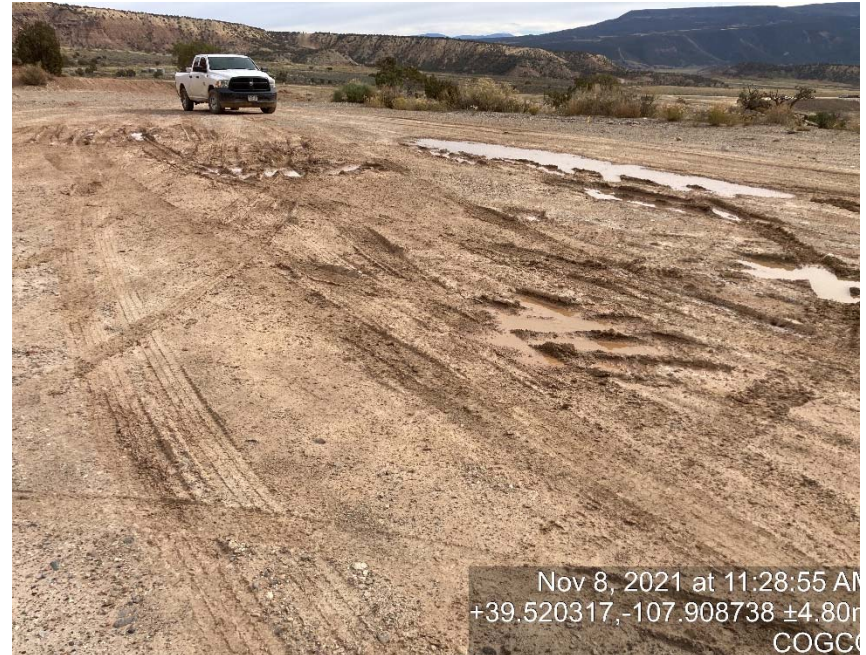
Lack of stabilization/ compaction
