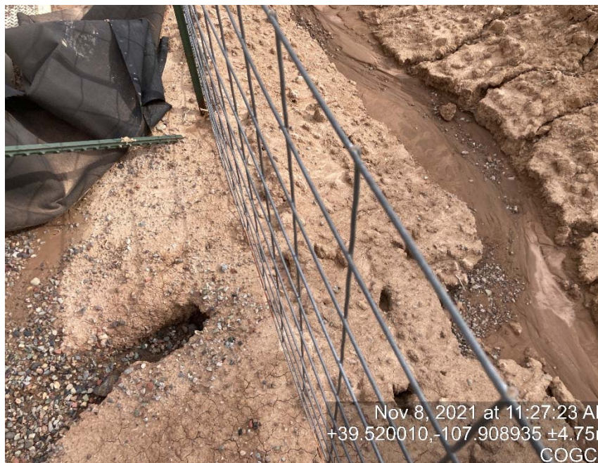
Tunneling through berm
