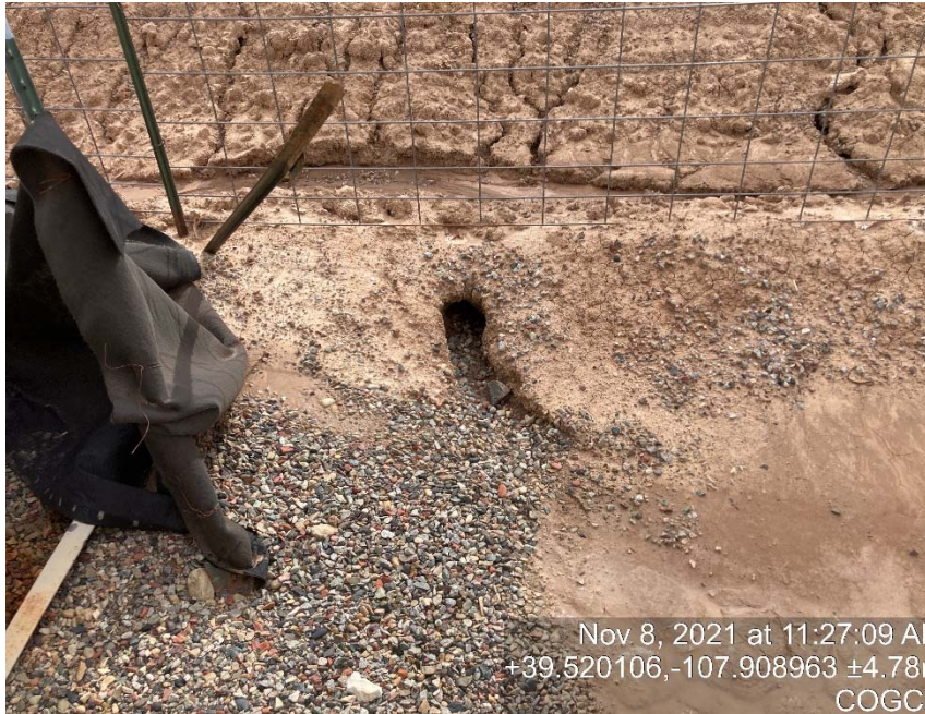
Tunneling through berm
