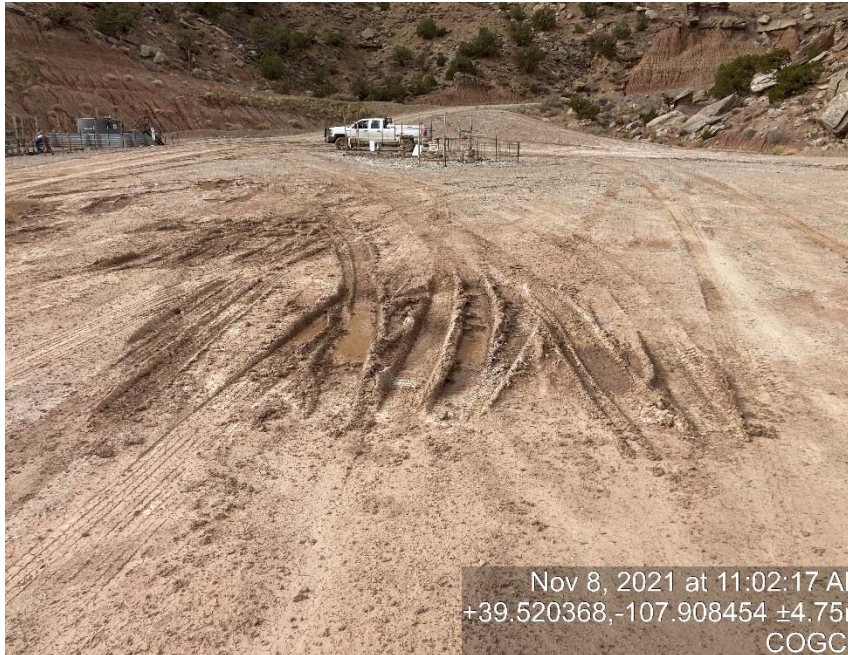
Lack of stabilization/ compaction
