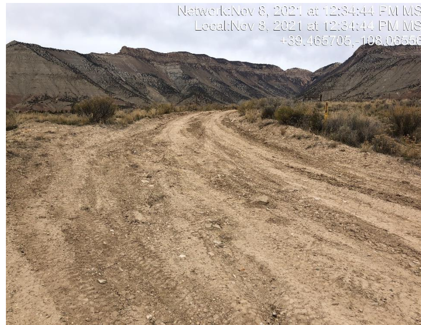
Photo #5173 Insufficient tracking BMP at entrance to location.
