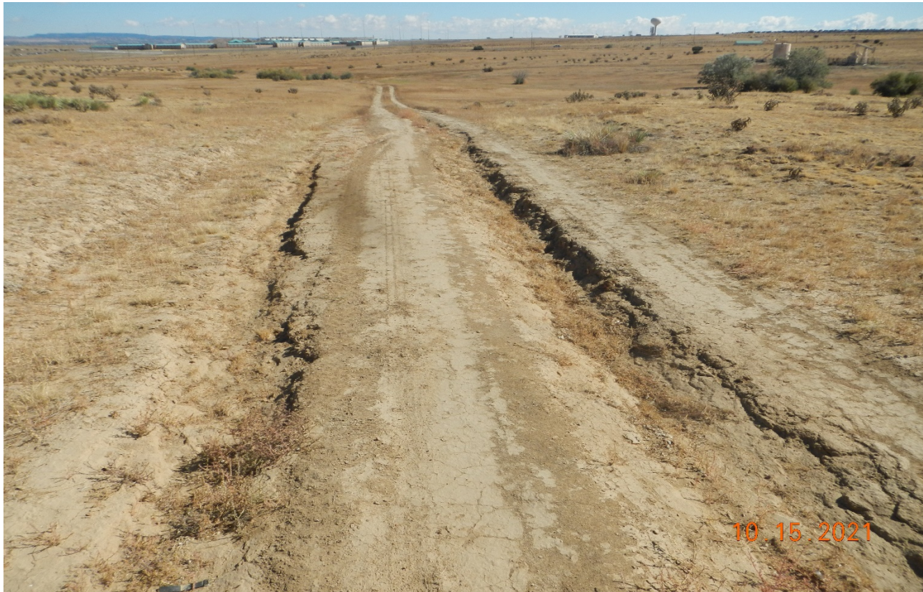
Photo 1. There is erosion along the access road that needs to be repaired and stabilized.
