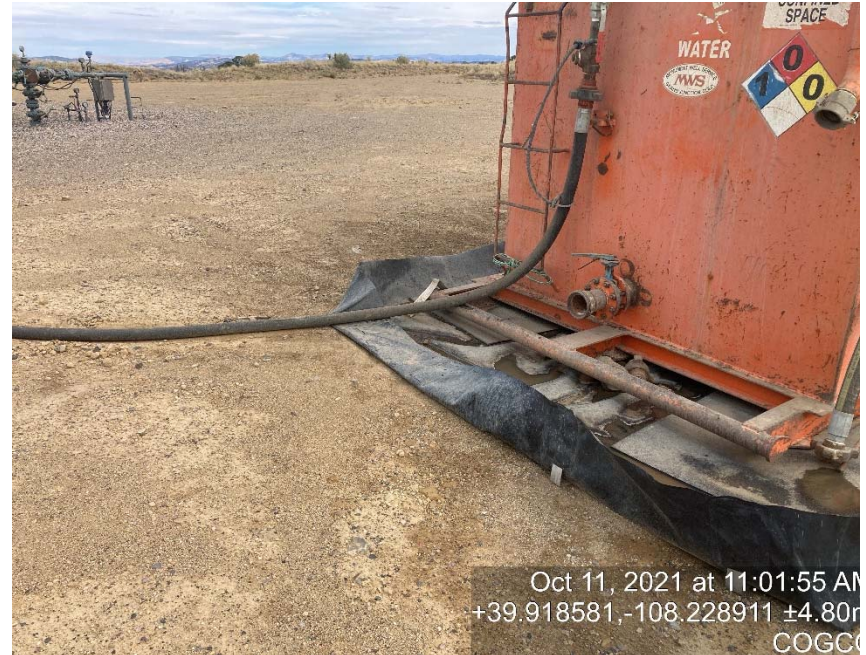
Lack of labeling/failing containment
