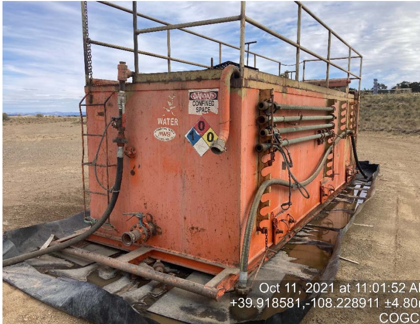
Lack of labeling/failing containment
