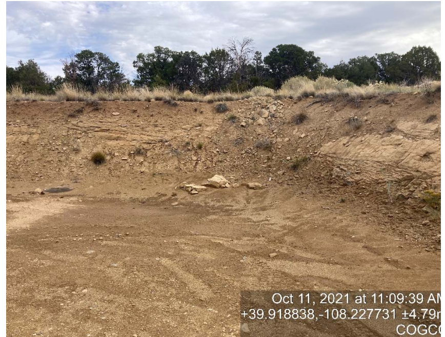
Lack of stabilization/erosion
