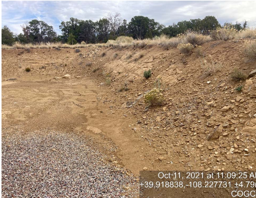
Lack of stabilization/erosion
