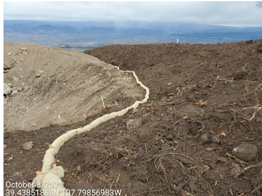
Photo 4: Photos taken from the topsoil stockpile on the west end of the Location. Erosion logs placed along perimeter of stockpile. Photos also show control measures to protect/stabilize the topsoil stockpile are missing or insufficient
