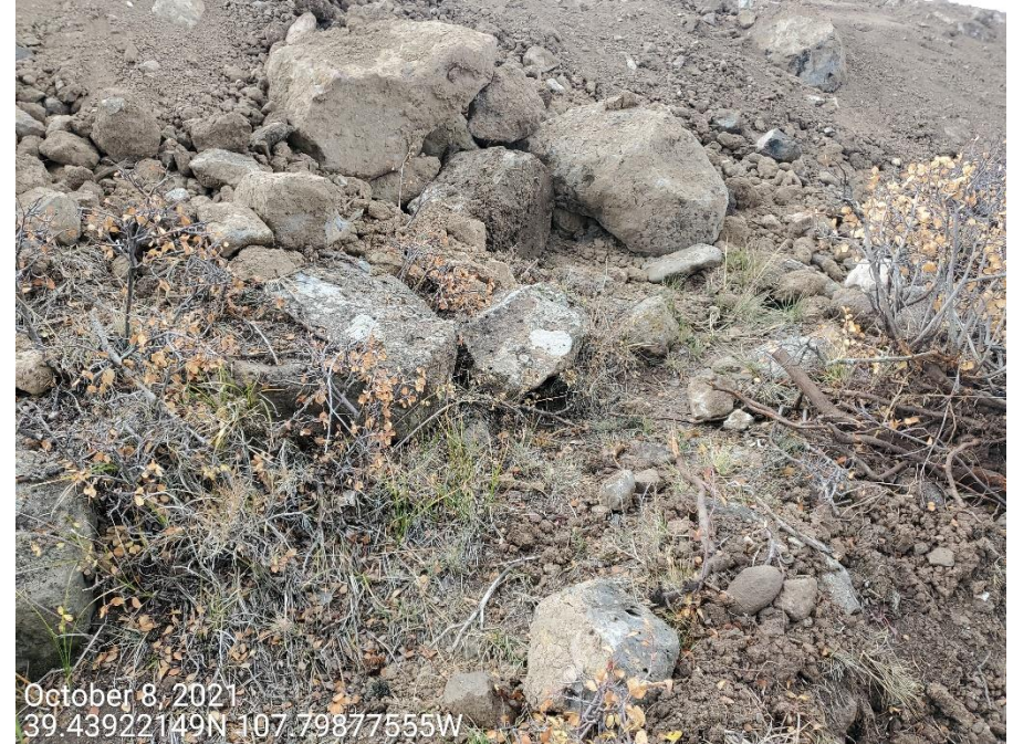
Photo 14: Photos taken from the fill slopes of the Location. Photos provide examples of areas observed where intact, rooted vegetation and topsoil can be observed beneath fill material; Operator failed to salvage, segregate and store all topsoil within the Location's disturbance area during construction.
