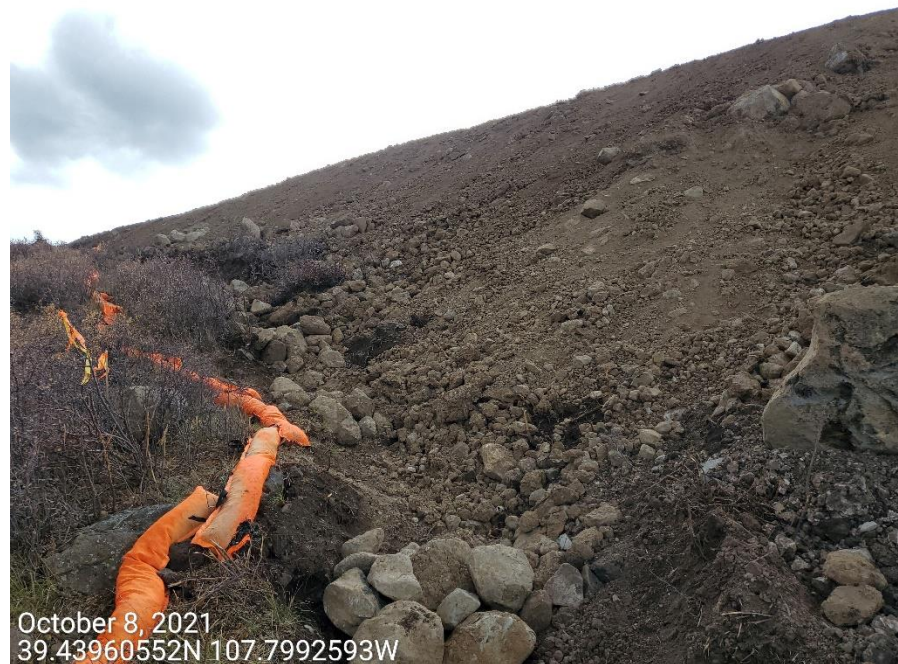
Photo 7: Photos provide examples of the fill slopes on the Location; stormwater and erosion control measures to protect/stabilize the fill slopes are missing or insufficient; slopes are loose/unconsolidated material
