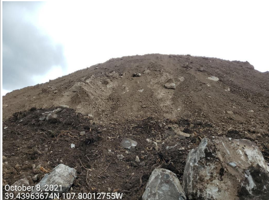
Photo 7: Photos provide examples of the fill slopes on the Location; stormwater and erosion control measures to protect/stabilize the fill slopes are missing or insufficient; slopes are loose/unconsolidated material
