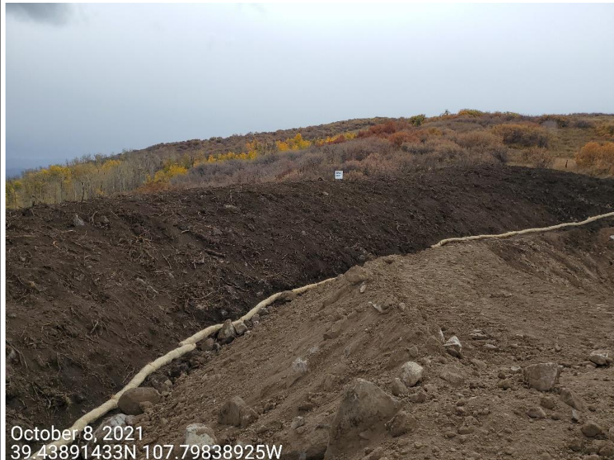
Photo 4: Photos taken from the topsoil stockpile on the west end of the Location. Erosion logs placed along perimeter of stockpile. Photos also show control measures to protect/stabilize the topsoil stockpile are missing or insufficient
