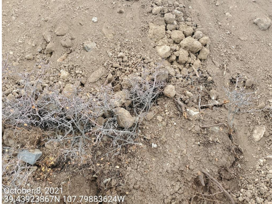
Photo 14: Photos taken from the fill slopes of the Location. Photos provide examples of areas observed where intact, rooted vegetation and topsoil can be observed beneath fill material; Operator failed to salvage, segregate and store all topsoil within the Location's disturbance area during construction.
