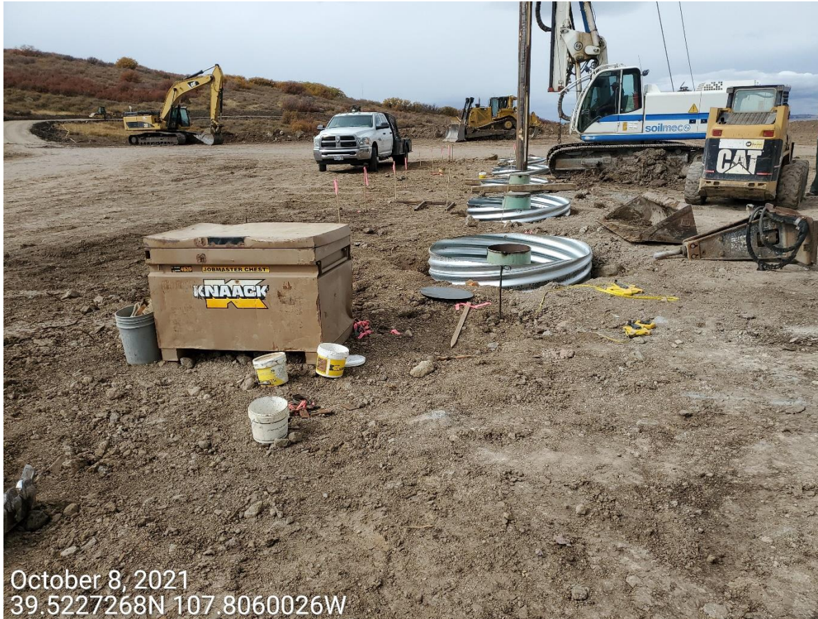
Photo 16: Photo taken from the Location. Photo shows Operator was in the process of drilling/installing conductor settings at time of inspection.
