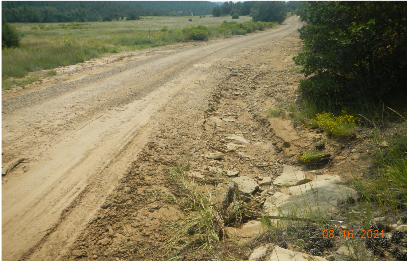
Photo 3. The same culvert inlet is filled in with sediment.
