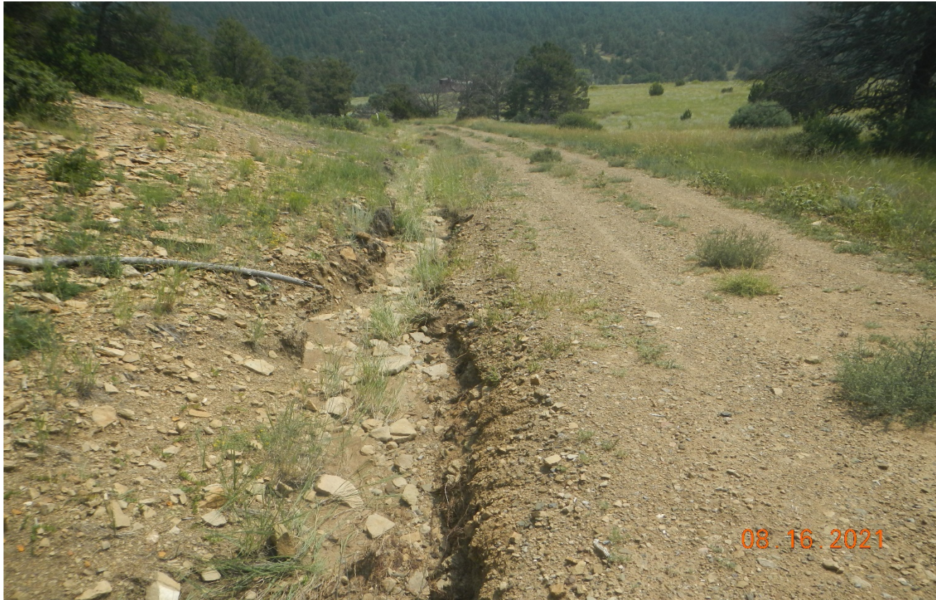
Photo 7. Facing back east along the access road. There is insufficient BMP's along this portion of the road.
