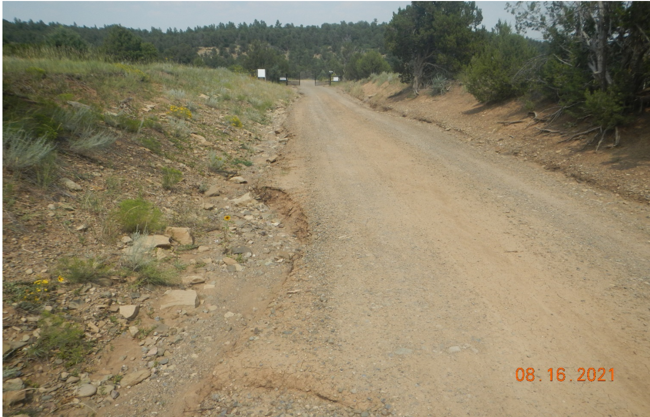
Photo 1. Facing northeast along the main road near the electric gate. Stormwater is directed down the road side in this area which is contributing to erosion of the county road.
