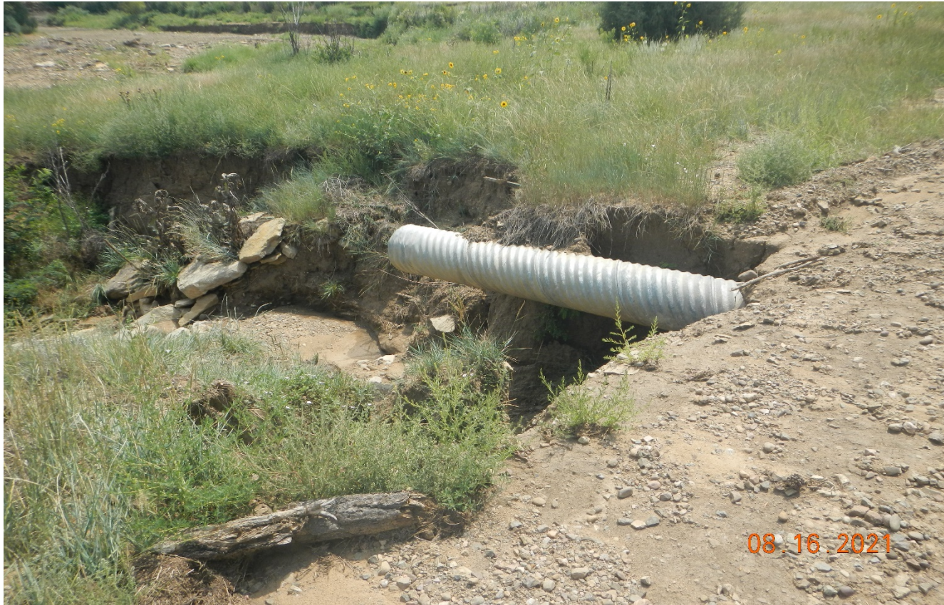
Photo 2. This culvert along the main road is partially washed out and needs to be repaired.
