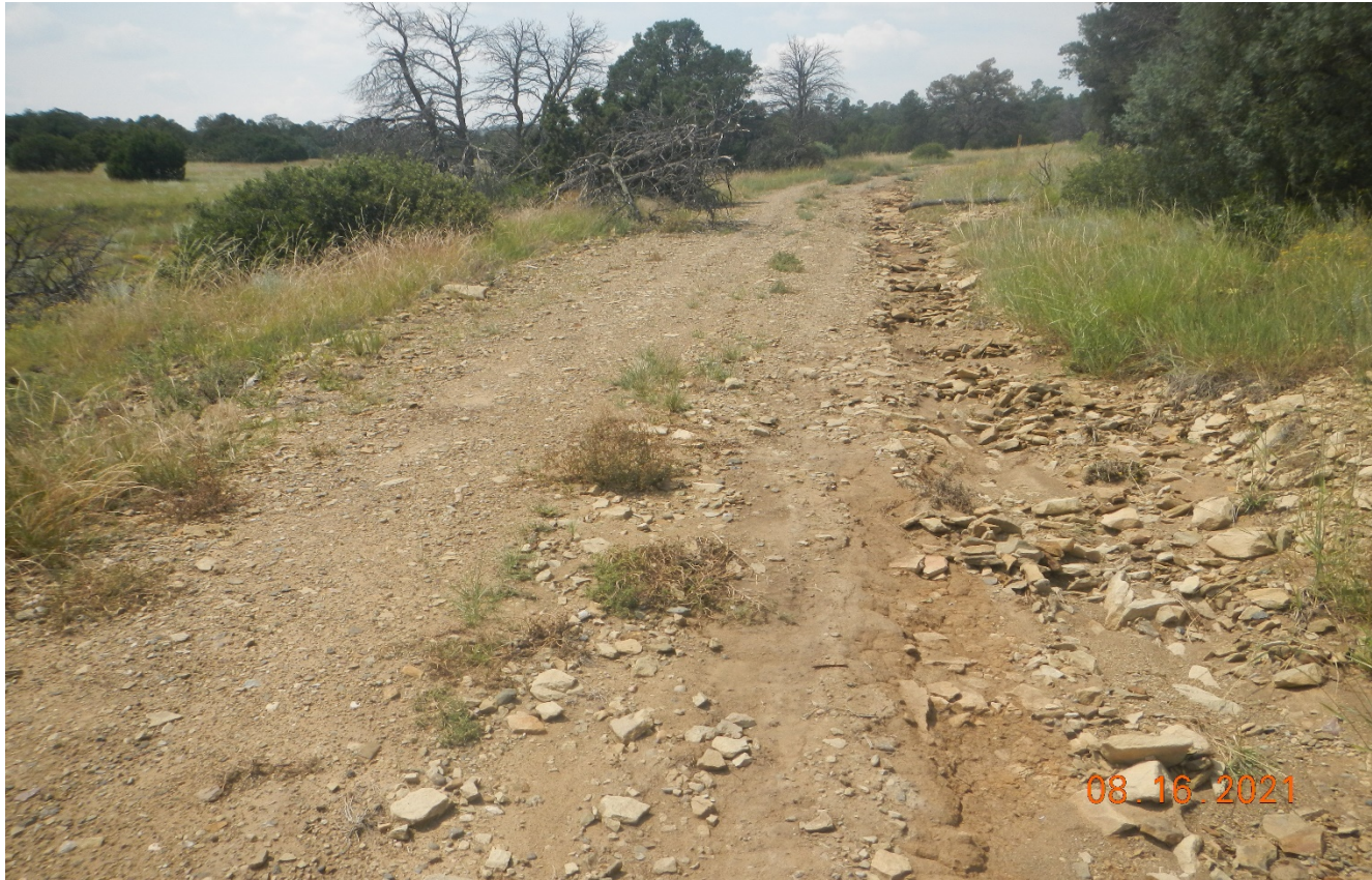
Photo 6. Further west along the access road there is erosion along the road. BMP's need to be installed along the road.
