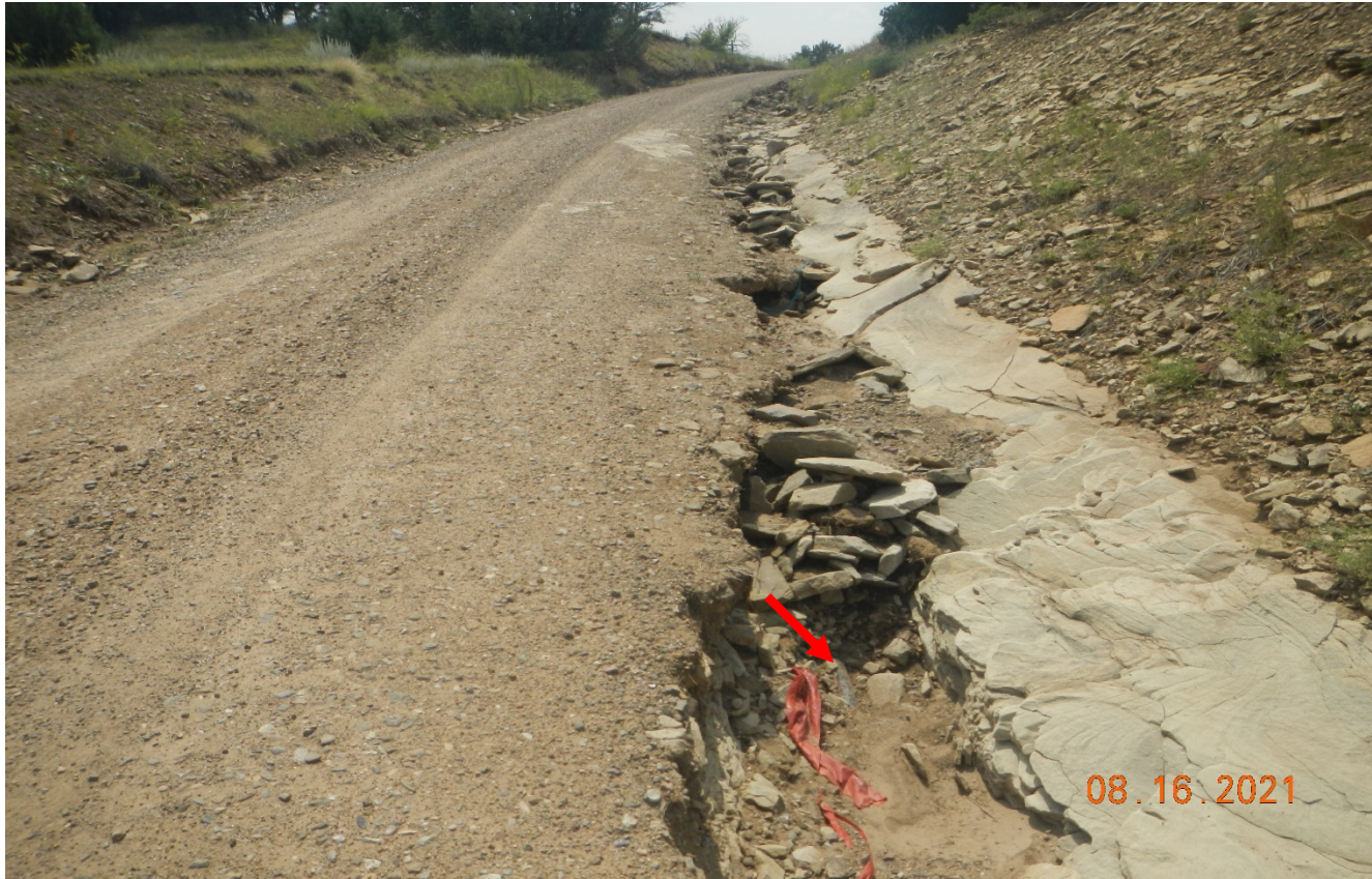
Photo 4. There is erosion along the side of the road which has exposed a pipe line shown at red arrow.
