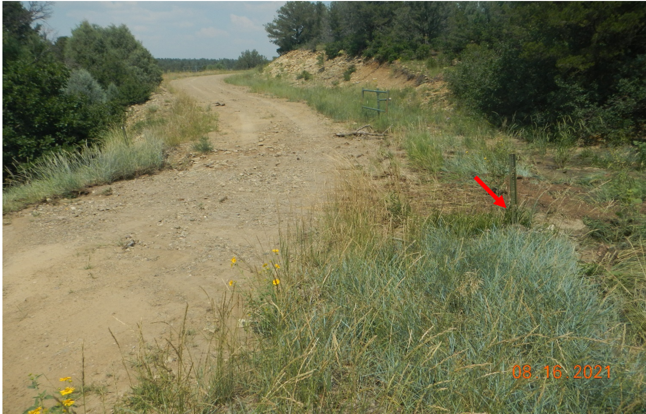
Photo 1. Facing northeast toward the access road. The culvert shown at red arrow is filled in with sediment. Stormwater flowed across the road in this area. The culvert will need to be repaired.
