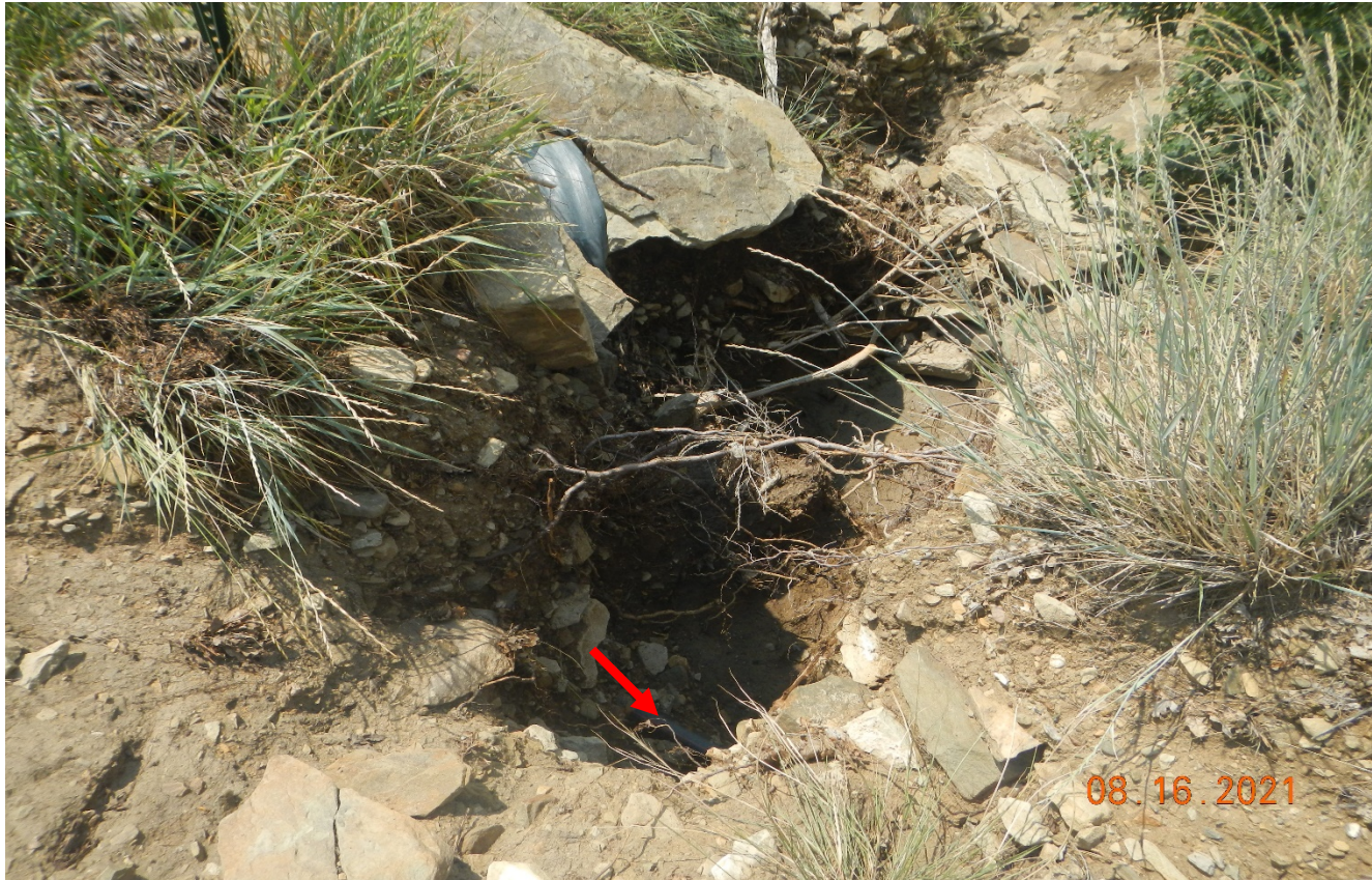
Photo 2. Erosion at the culvert outlet has exposed the pipe line shown at red arrow. This area will need to be repaired.
