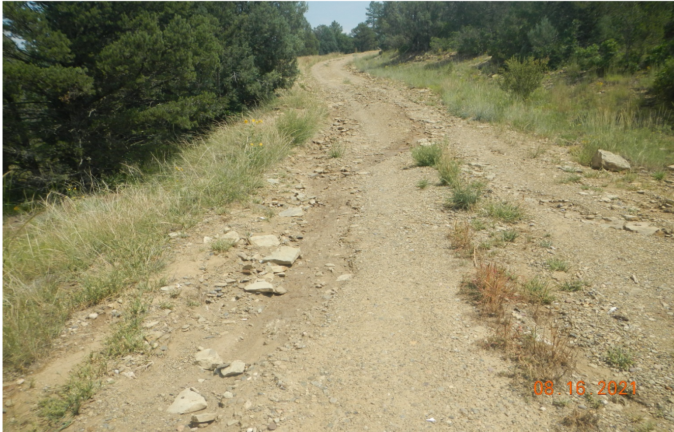
Photo 3. Stormwater erosion is occurring down the road. The road will need to be graded and repaired.
