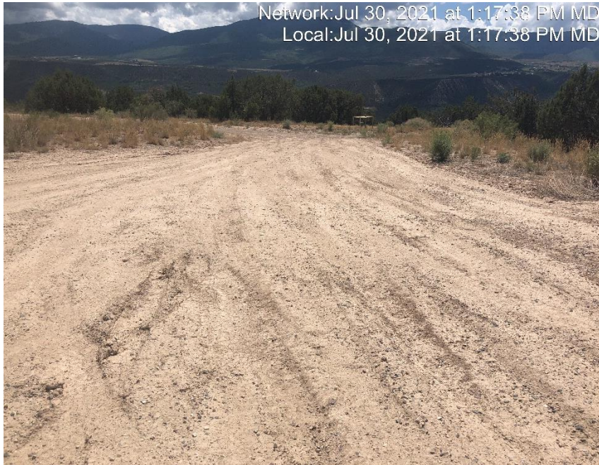
Photo #4638 Location lacks stabilization.
