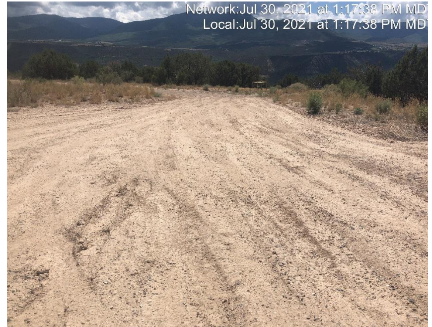
Photo #4638 No form of tracking BMP located at entrance to location.
