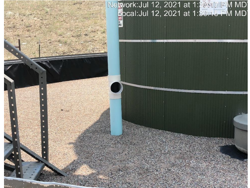
Photo #4388 Heating insulation open ended and not capped.
