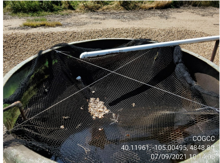
Photo 6 Open top partially buried produced water vessel
