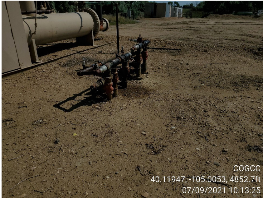
Photo 5 Leaky header
