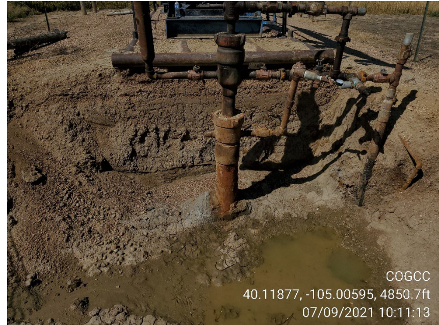
Photo 2 Excavation at well, water in bottom of excavation, weeping well casing
