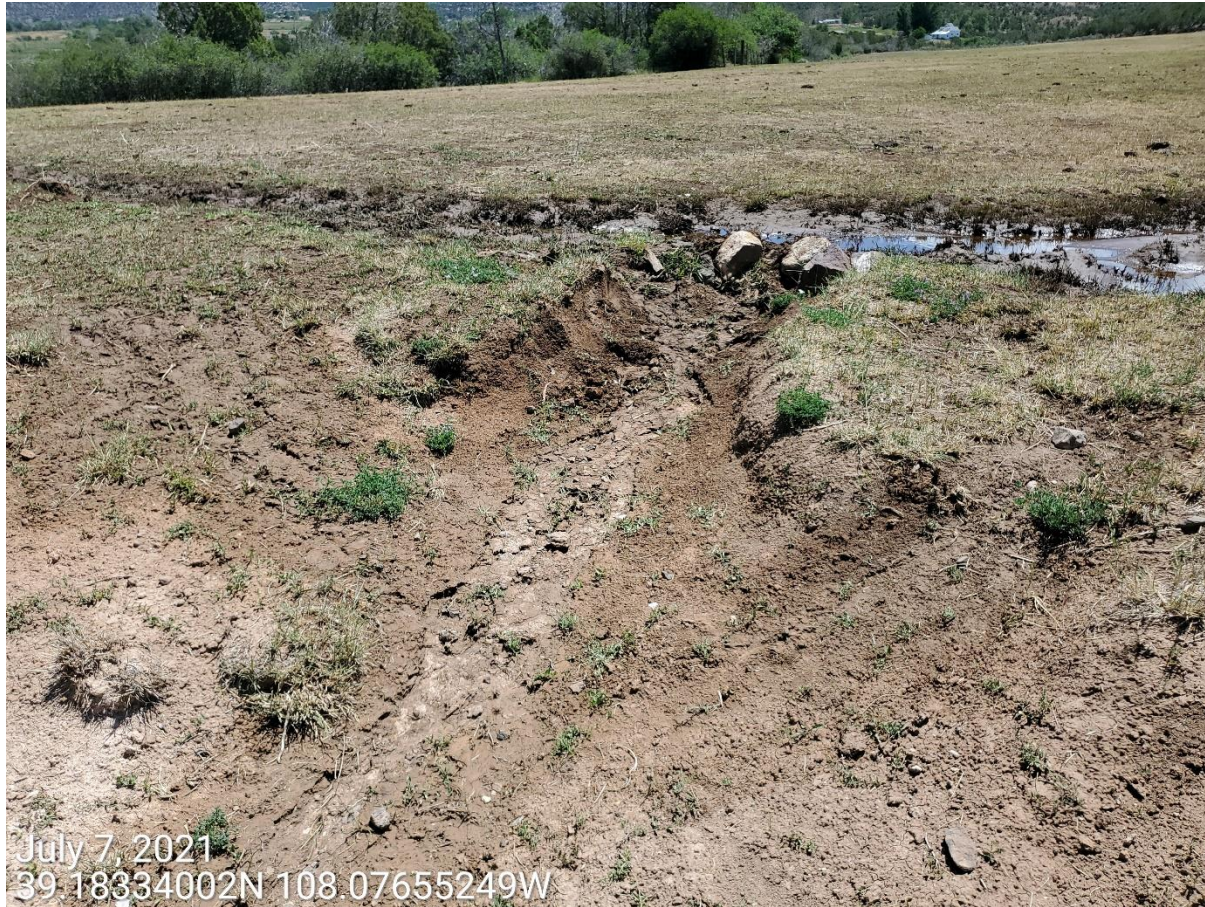
Photo 4: Photo taken from the cut slopes on the southeast end of the Location. Photo shows erosion degradation observed on the slopes.
