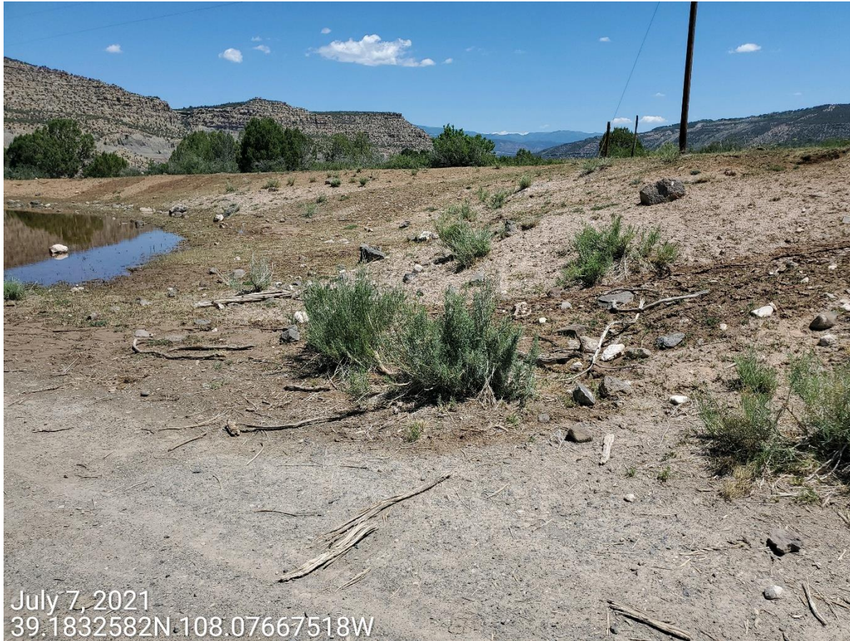
Photo 3: Photo taken from the southeast end of the Location, facing northeast. Photo shows cut slopes and edge of the pad.
