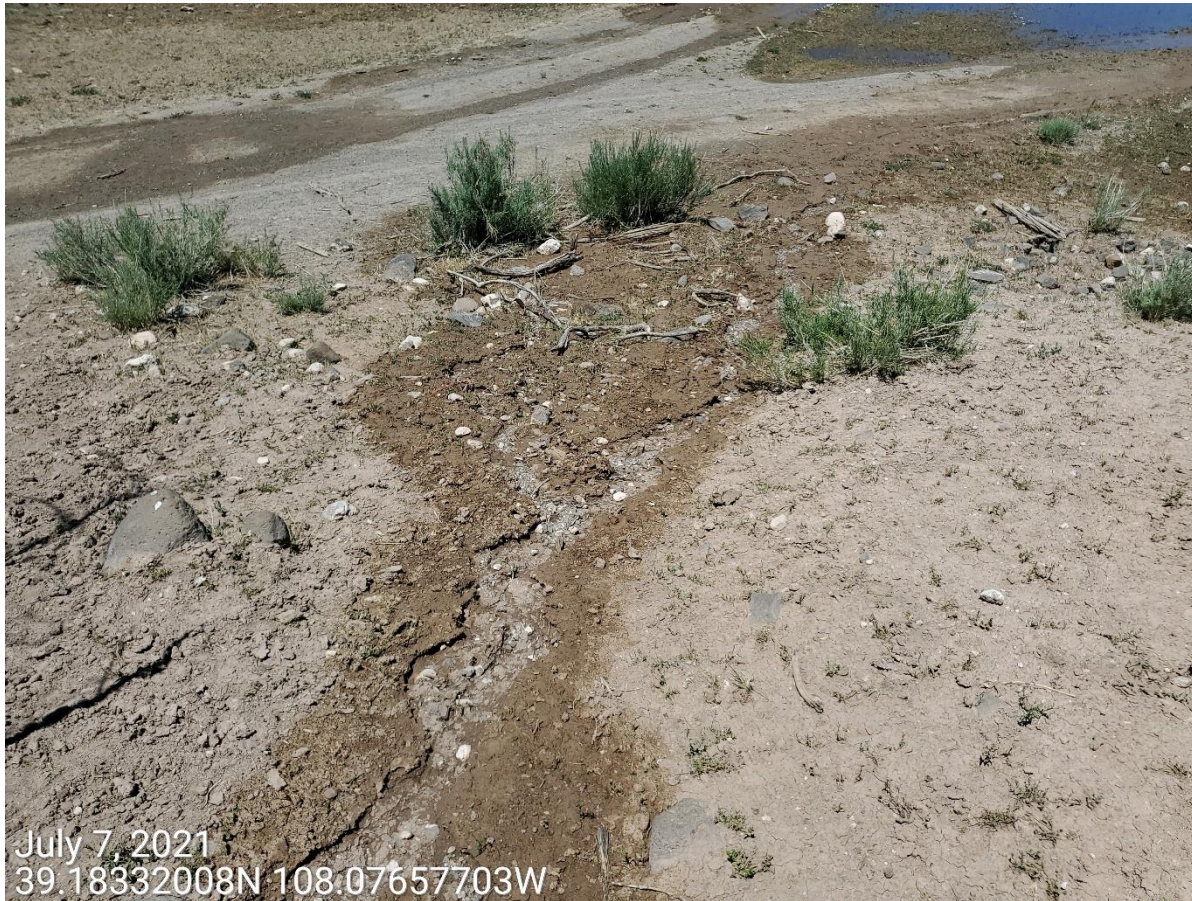
Photo 6: Photo taken from the cut slopes on the southeast end of the Location. Photo shows erosion degradation observed on the slopes.
