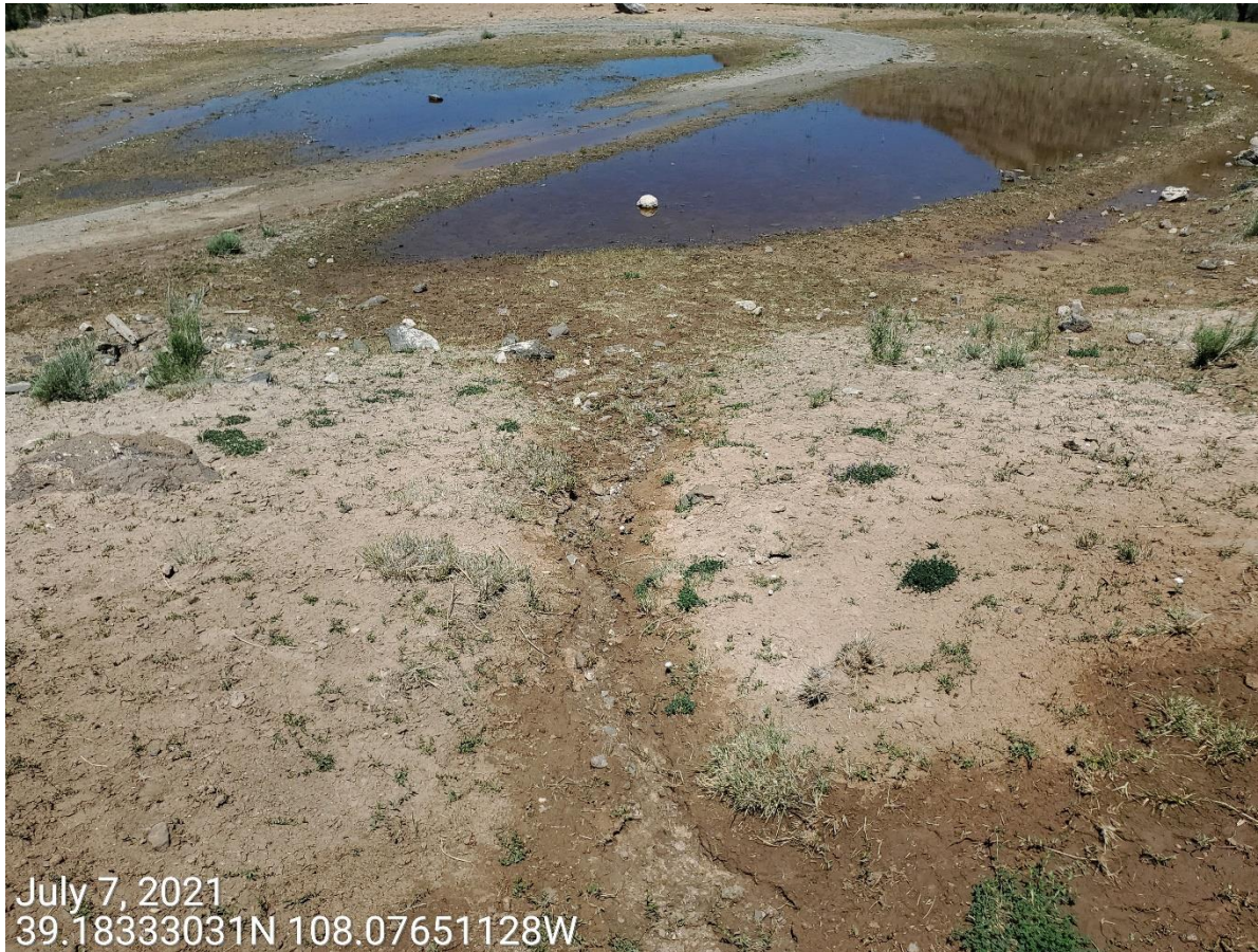
Photo 5: Photo taken from the cut slopes on the southeast end of the Location. Photo shows erosion degradation observed on the slopes.
