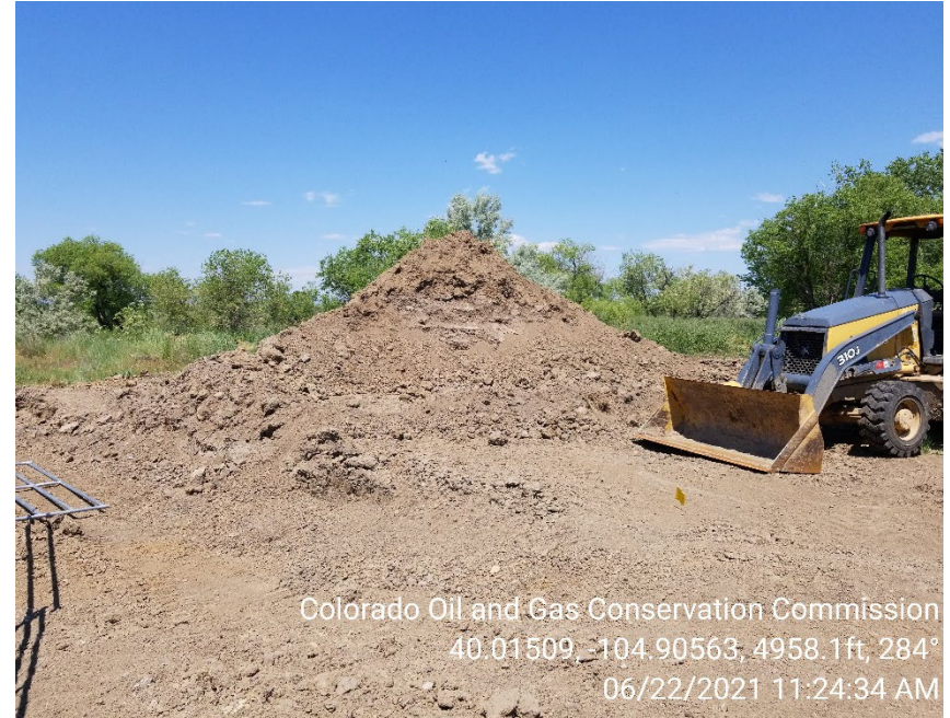
Photo 8 – Soils stockpiled on location with inadequate BMPs.
