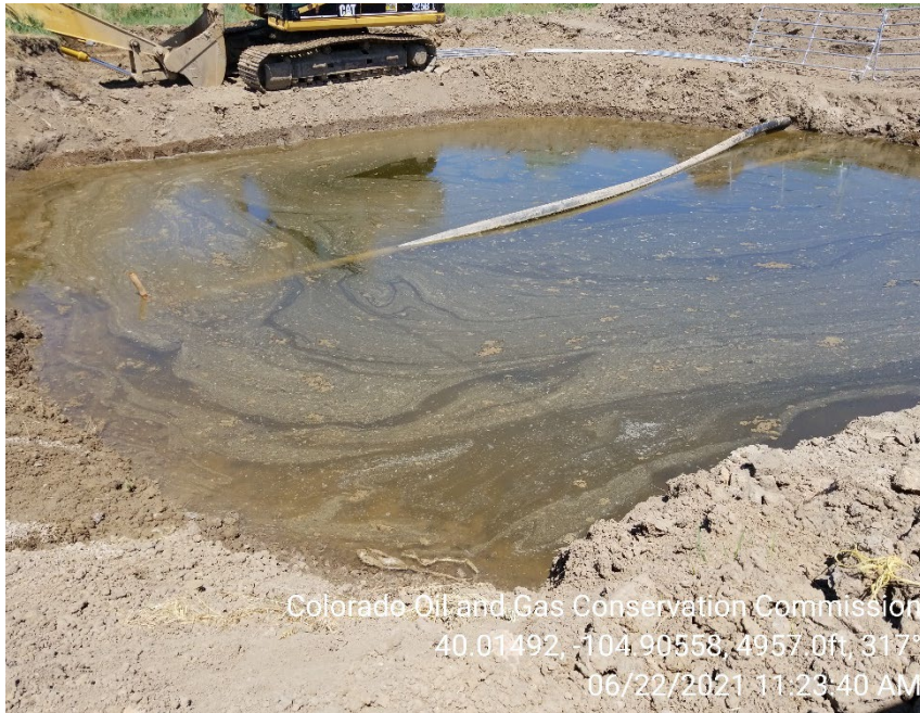
Photo 5 – Open excavation. Hydrocarbon sheen observed on groundwater.
