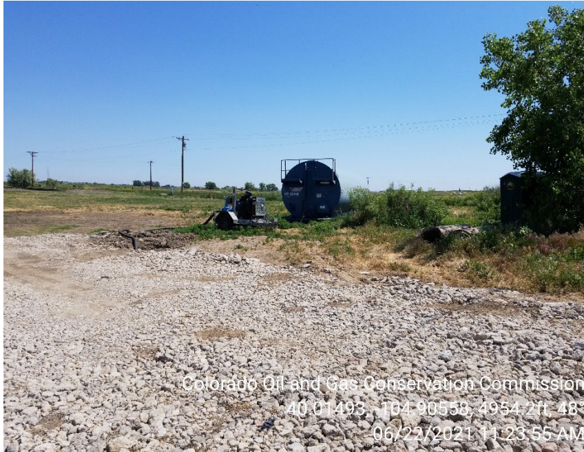
Photo 7 – Groundwater removed from open excavation being stored on site.
