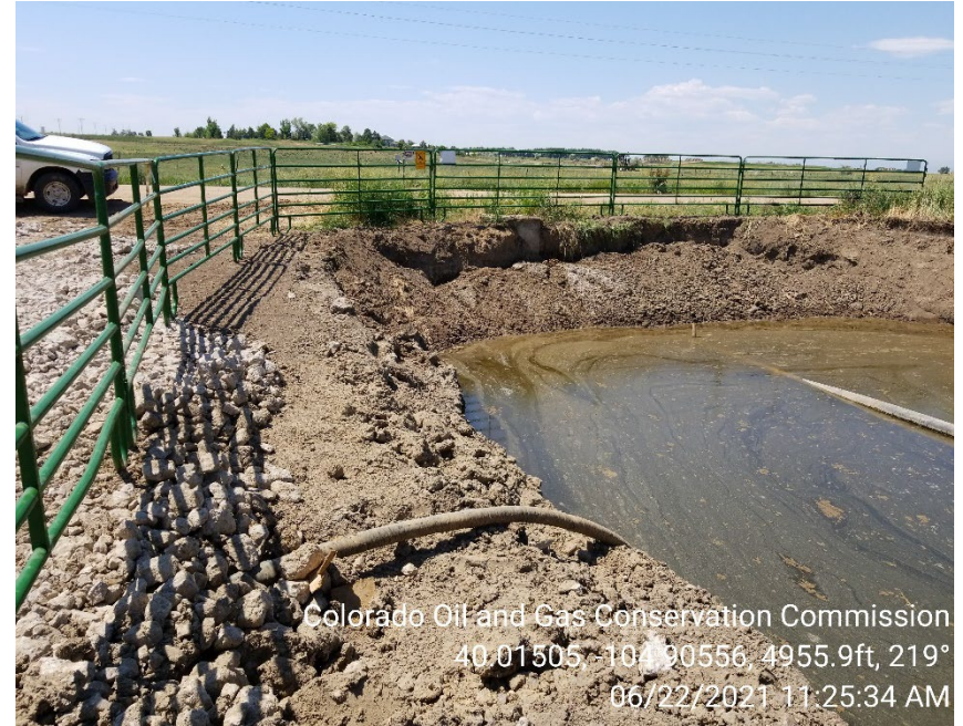
Photo 2 – Open excavation with groundwater. Impacts appear to remain in situ in southern wall.
