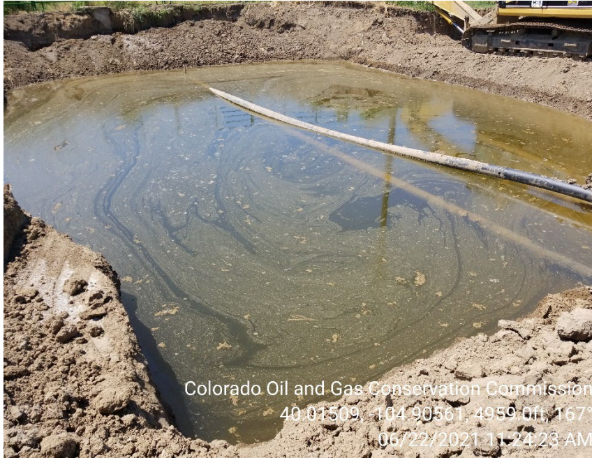
Photo 3 – Open excavation. Hydrocarbon sheen observed on groundwater.
