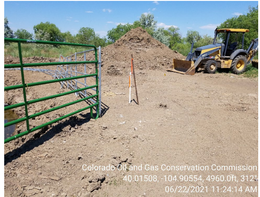
Photo 6 – One monitoring well installed outside of open excavation.
