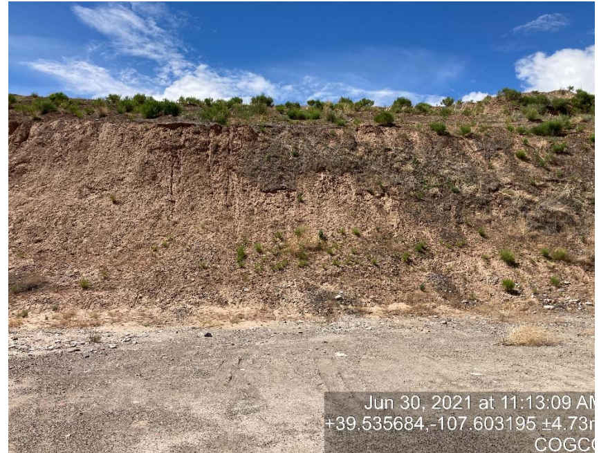
Lack of stabilization/erosion on cut slope
