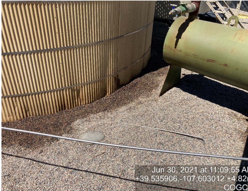
Staining all the way around condensate tank
