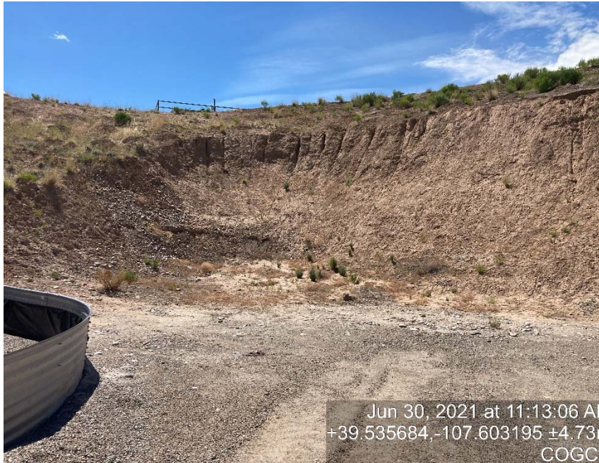
Lack of stabilization/erosion on cut slope
