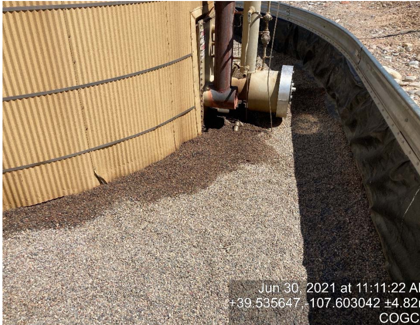
Staining all the way around condensate tank
