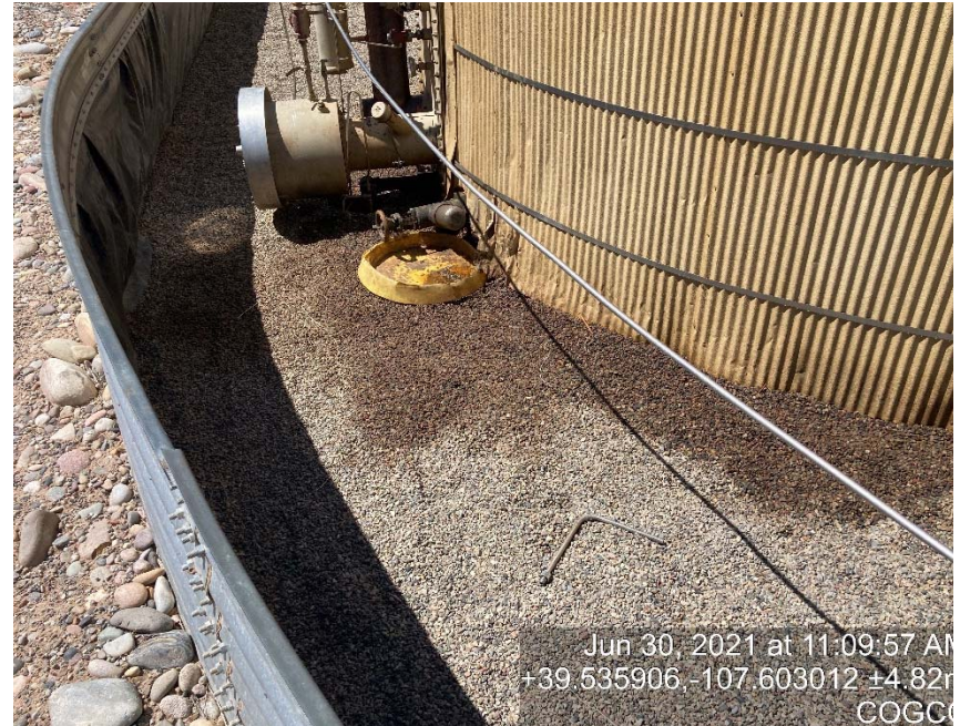
Staining all the way around condensate tank
