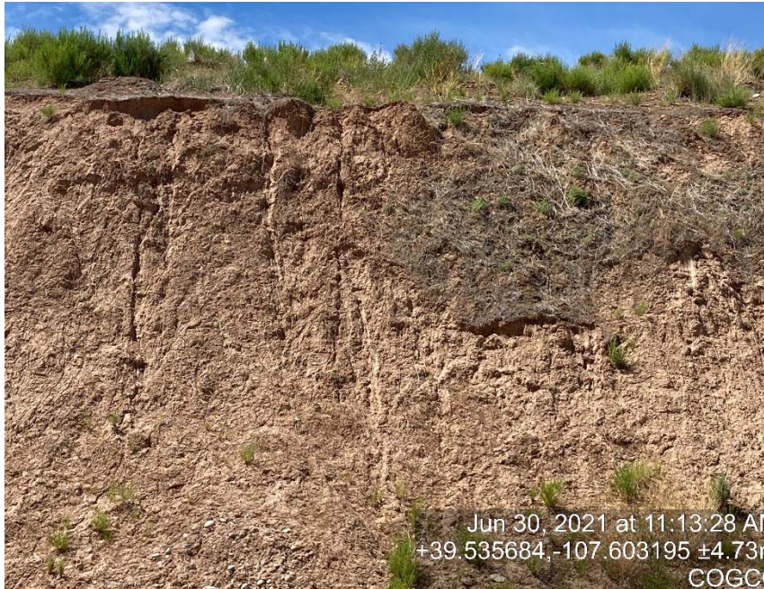
Lack of stabilization/erosion on cut slope
