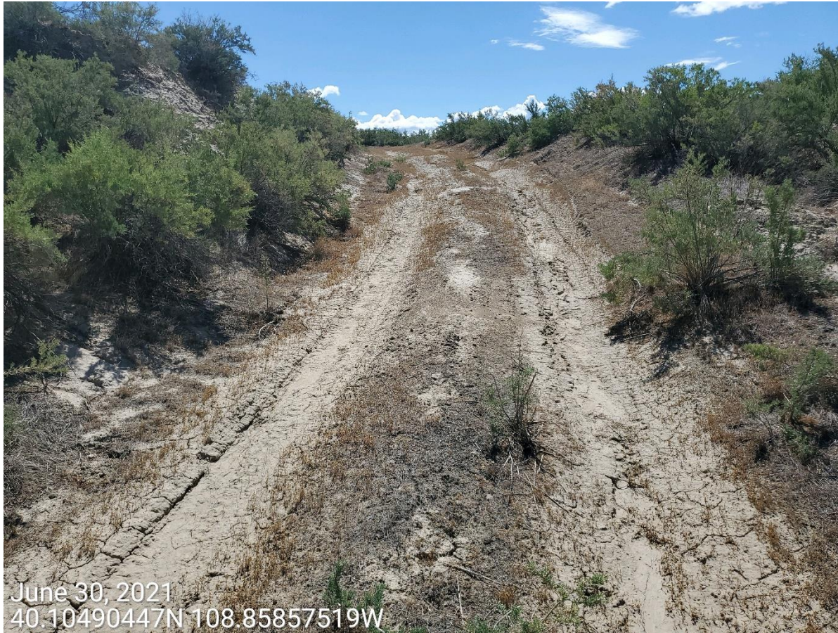
Photo 12: Photo taken from the southern access road, facing southeast. Compaction alleviation, recontouring and revegetation activities not performed.
