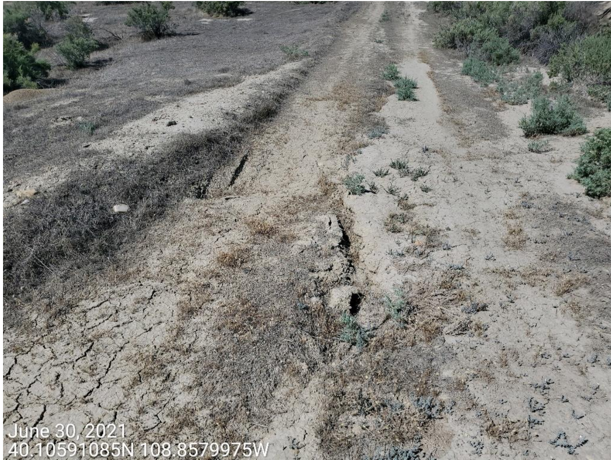
Photo 4: Photo taken along the access road. Photo shows erosion degradation.
