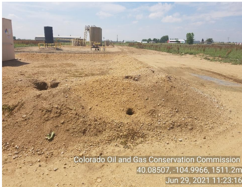
Photo 3 Berms have holes and are in disrepair.
