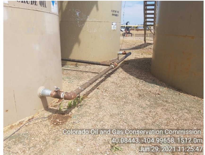
Photo 8 Stained soil under crude oil load lines.
