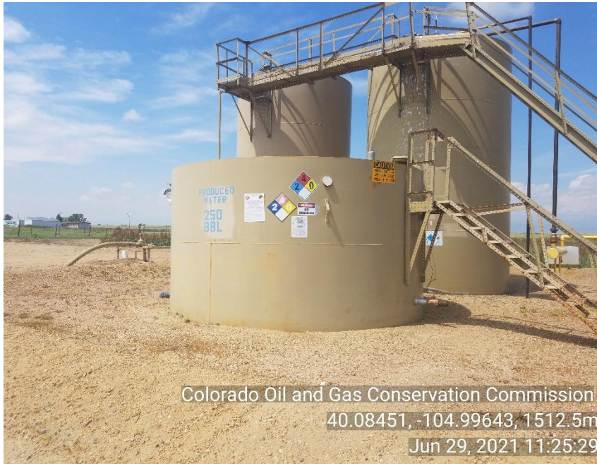
Photo 7 produced water tank
