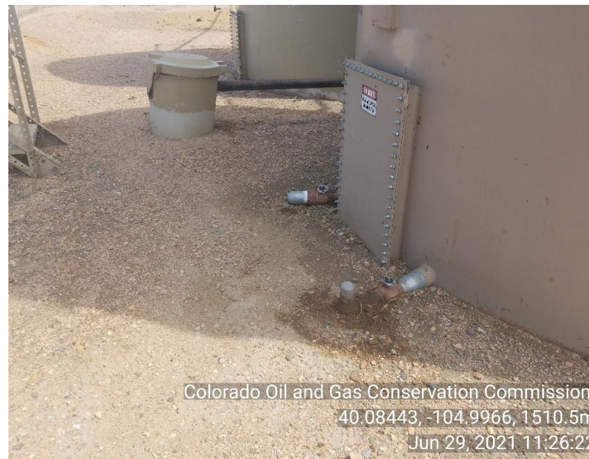
Photo 10 Stained soil and Mechanical issues Crude oil load lines.
