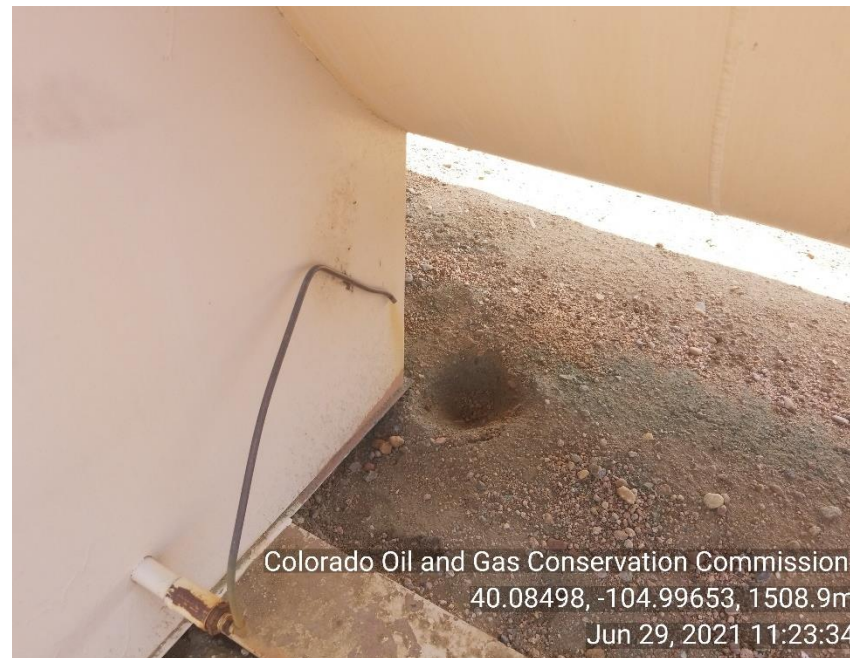
Photo 4 draining separator on ground.
