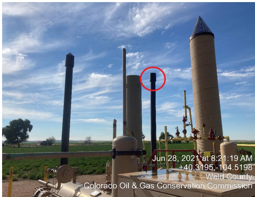
Photo #3 Missing Bird protector
