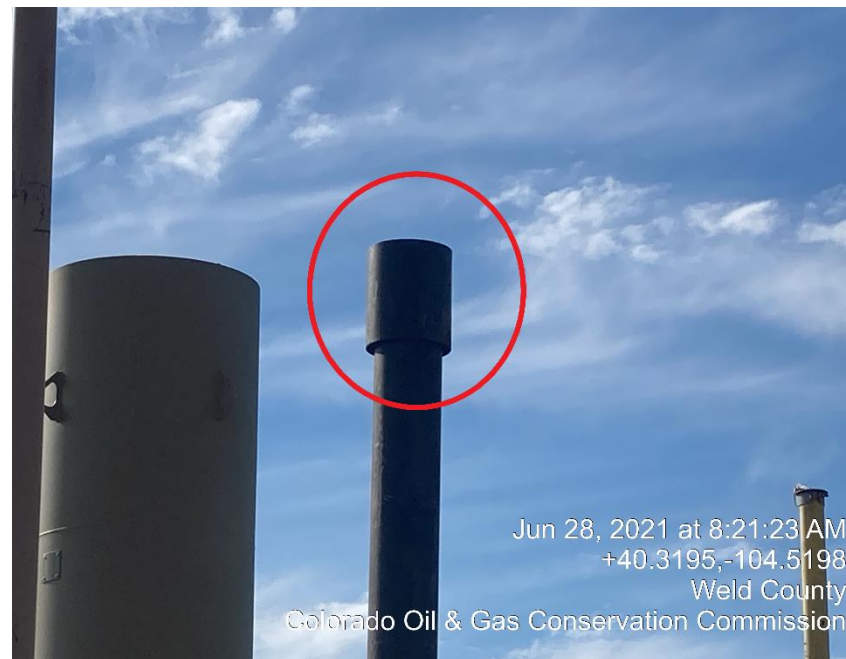
Photo #4 Missing Bird protector
