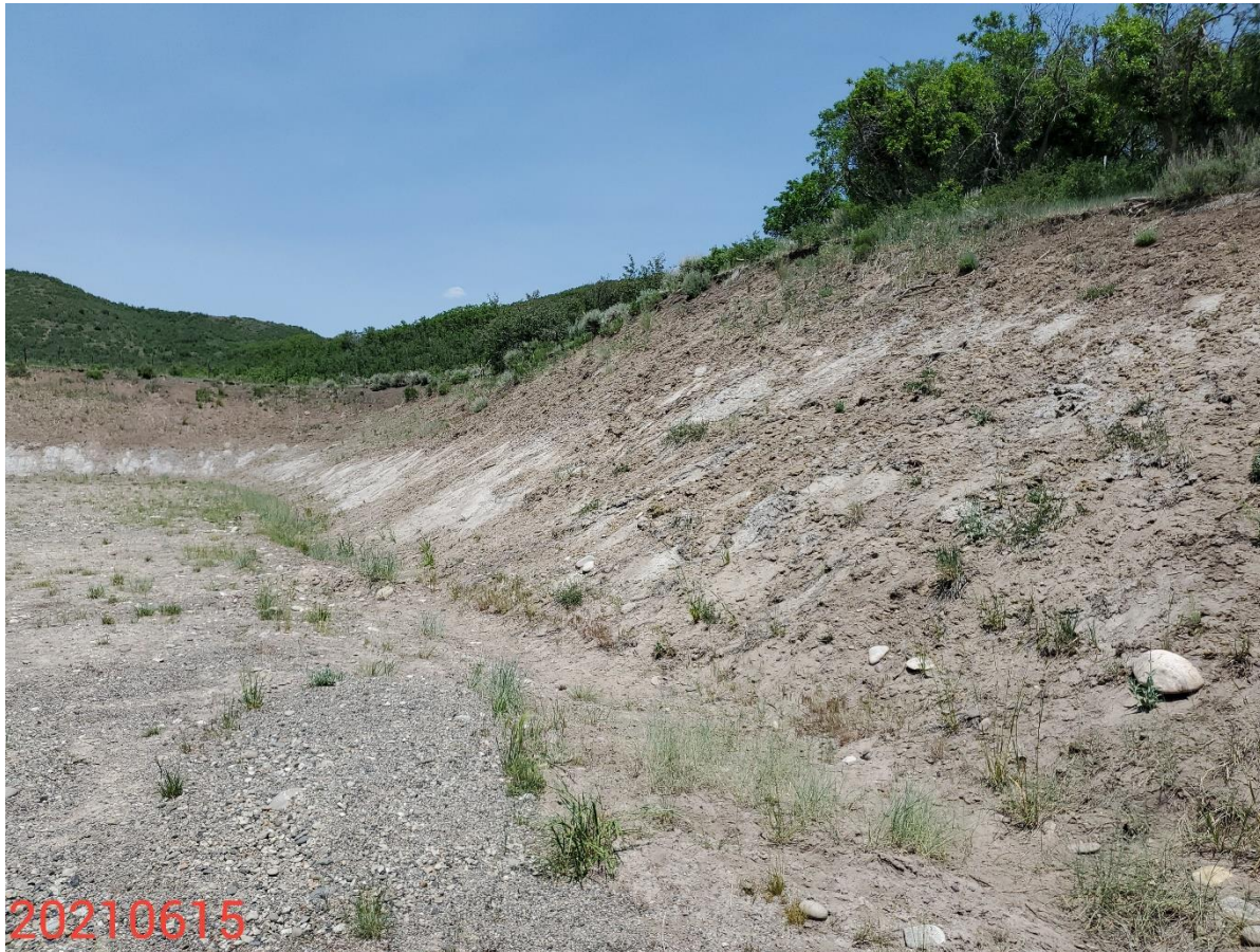
Photo 6: Photo taken from the cut-slopes on the southeast corner of the Location, facing north. Photo shows control measures (short term and long term) control measures to protect and stabilize the cut-slopes remain missing or insufficient.
