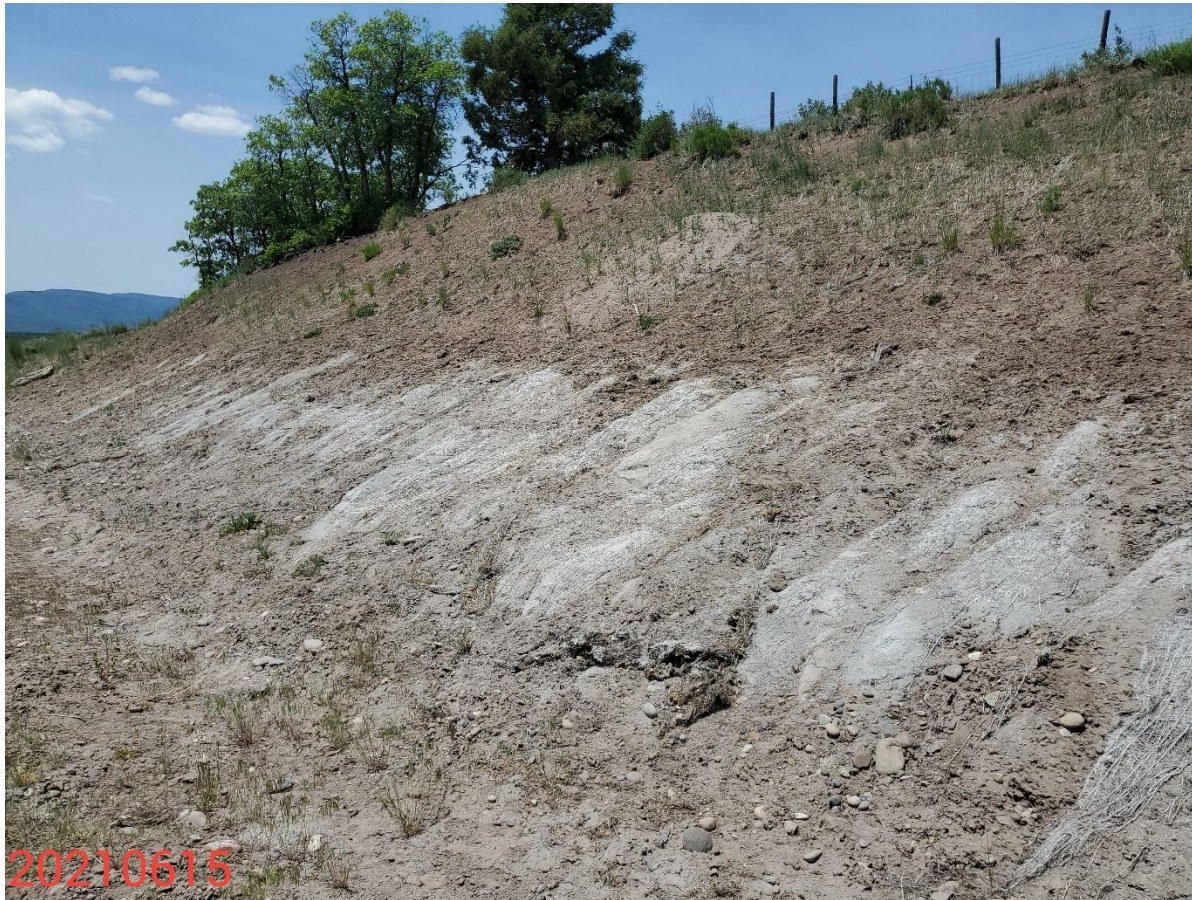
Photo 4: Photo taken from the cut-slopes on the northeast corner of the Location, facing west. Photo shows control measures (short term and long term) control measures to protect and stabilize the cut-slopes remain missing or insufficient.
