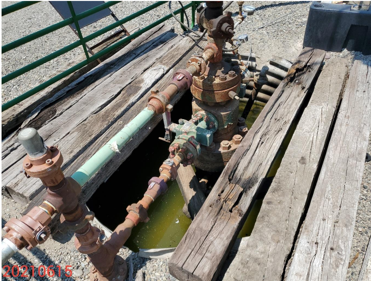
Photo 7: Photo off wellhead and cellar. Photo shows control measures to prevent wildlife access to the cellar, and to protect wildlife resources remain missing or inadequate. Photo also shows fluids/chemicals within cellar have not been removed.
