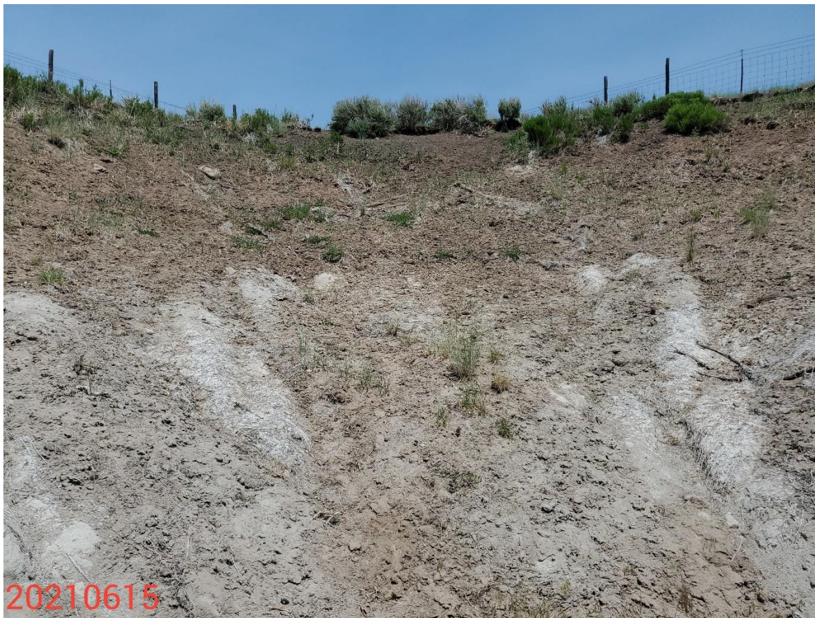
Photo 5: Photo taken from the cut-slopes on the northeast corner of the Location, facing northeast. Photo shows control measures (short term and long term) control measures to protect and stabilize the cut-slopes remain missing or insufficient.
