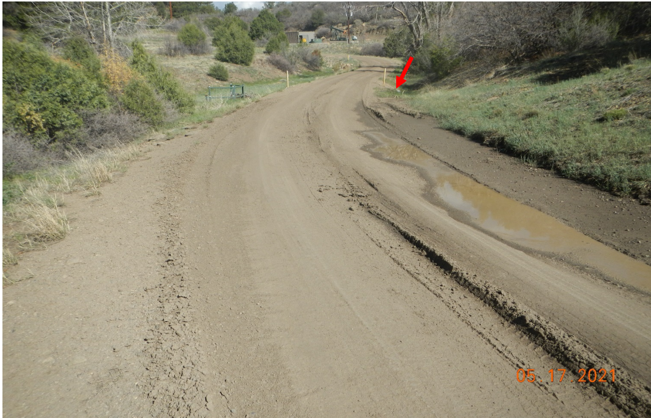
Photo 2. Stormwater is not directed toward the culvert (at red arrow) causing stormwater to accumulate on the road. Areas of rutting need to be stabilized.
