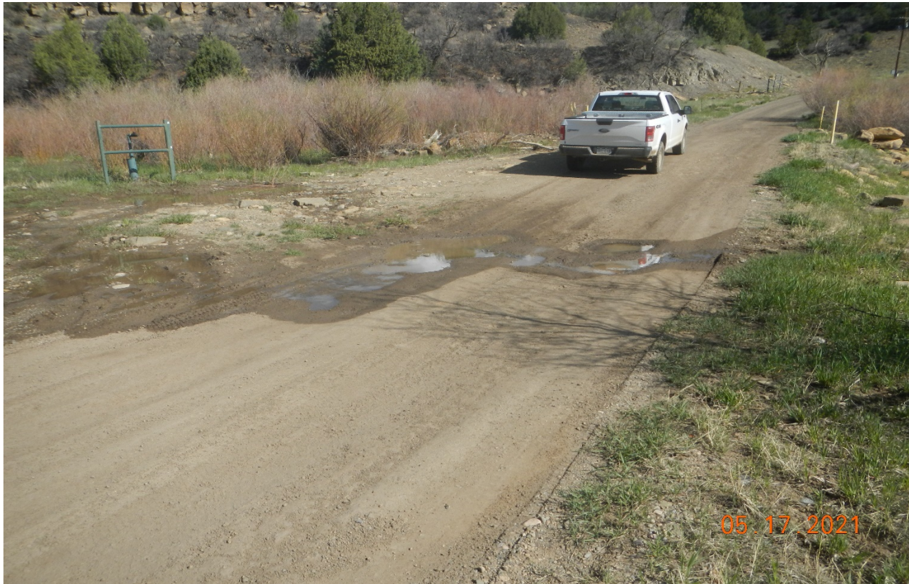
Photo 1. There is water from the river pooling onto the road in this area. BMP's need to be installed to prevent erosion of this area. E.G. Berm. Diversion ditch, culvert ect.
