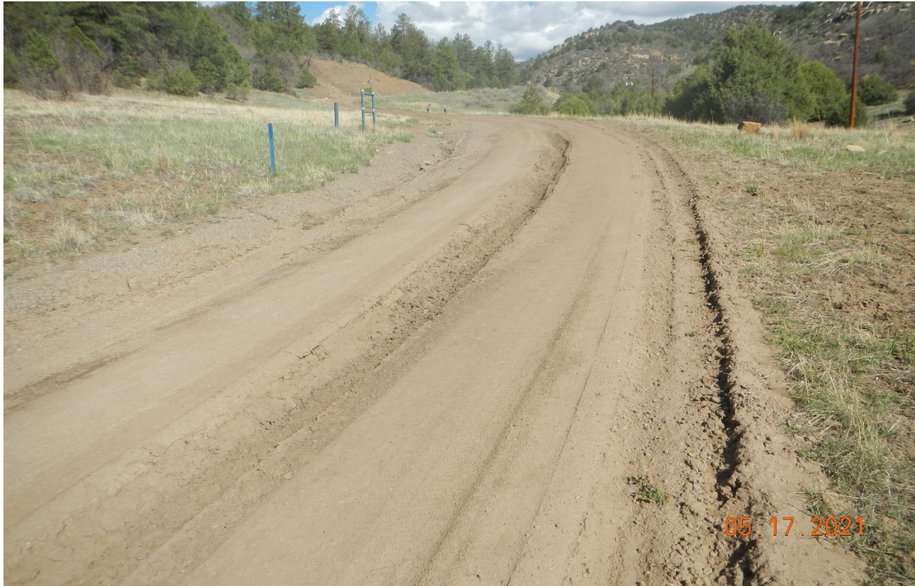
Photo 3. There is vehicle rutting along the main road. Areas of rutting need to be stabilized.
