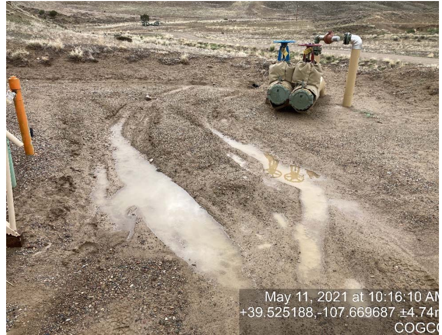
Lack of stabilization/compaction/drain
