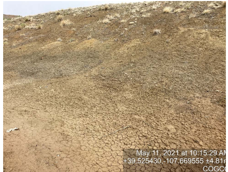
cut slope not stabilized
