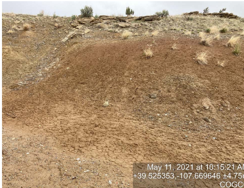
cut slope not stabilized
