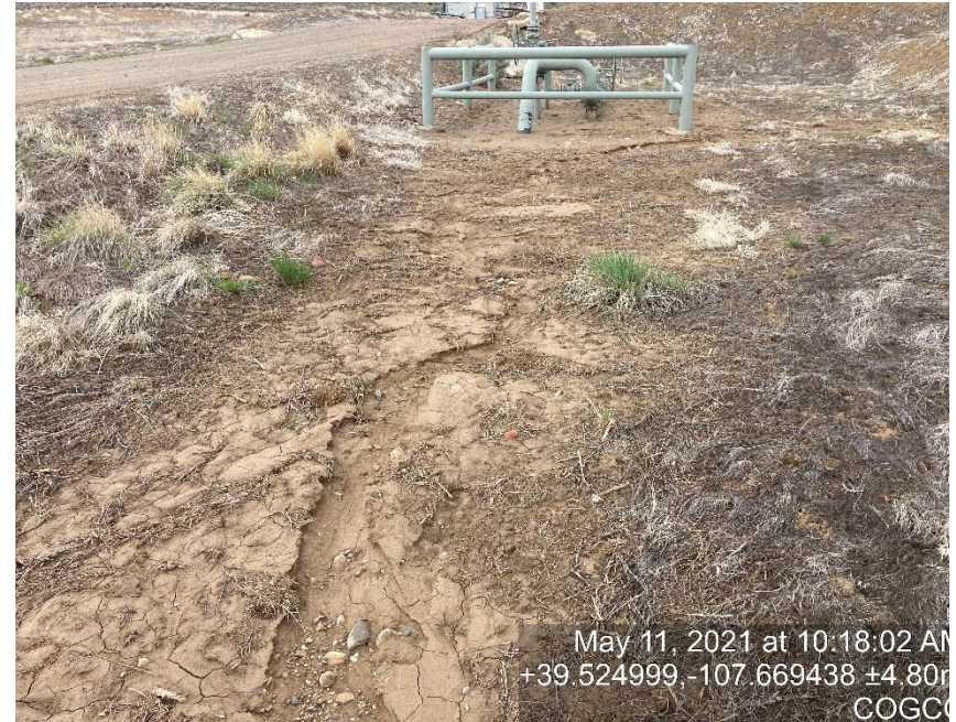
Sediment migration from drain on edge of location
