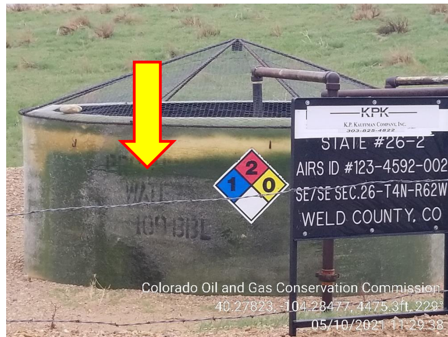
Photo 4 – Tank Battery Sign. Produced Water Label Weathered
