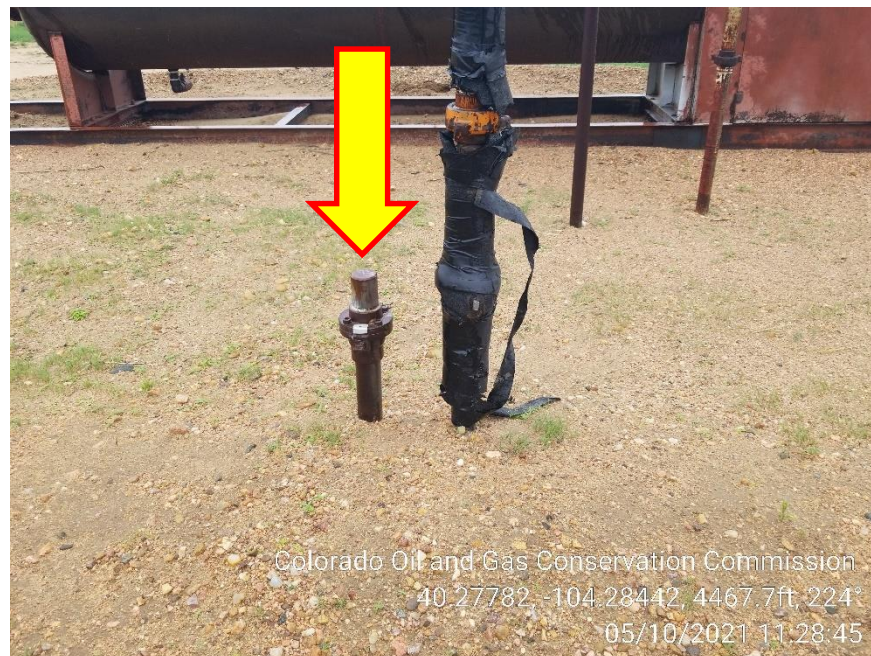
Photo 6 – Unmarked Riser at Separator
