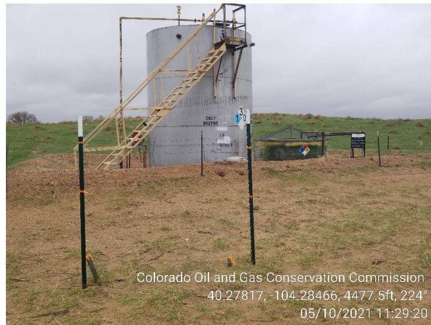
Photo 2 – Tank Battery, Deadman Anchors now Marked
