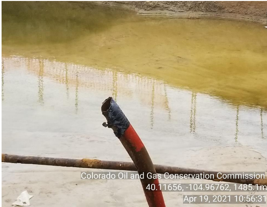
Photo 27 open ended pipe in open excavation.
