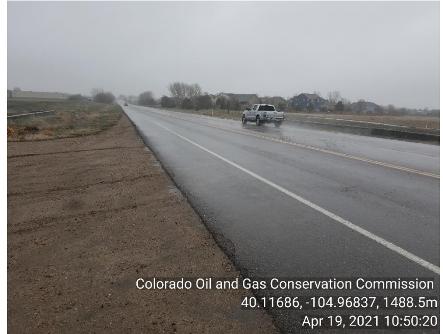
Photo 2 No tracking pad BMP on entrance # 1
