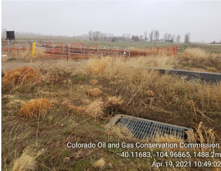
Photo 3 No inlet protection around storm drain.
