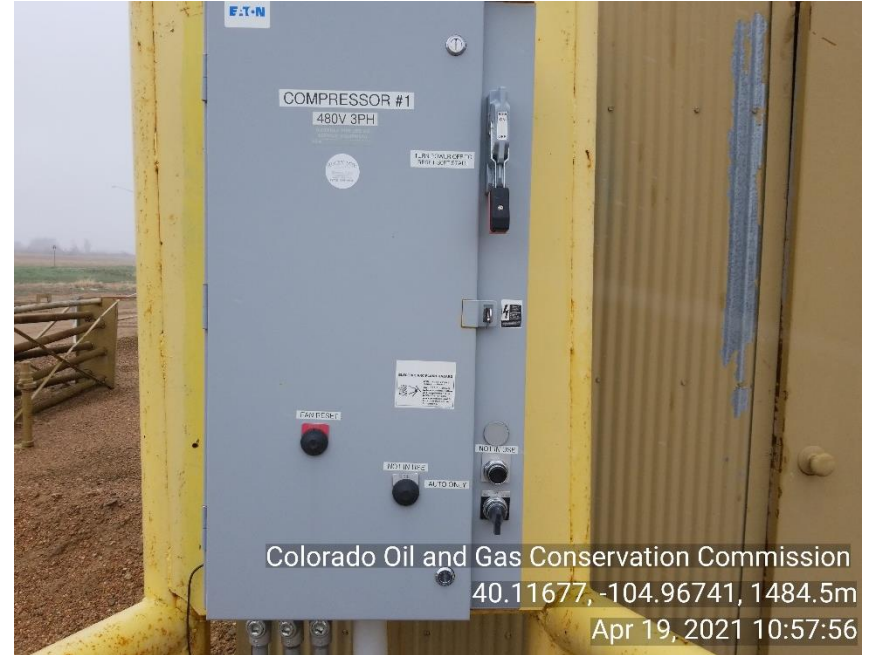
Photo 33 Compressor breaker box not LOTO accessible to the public.
