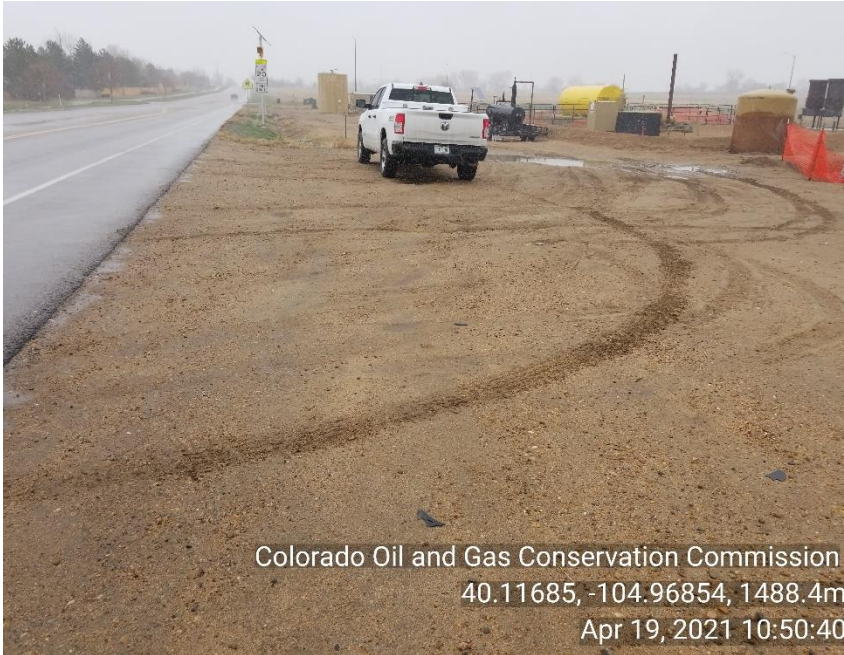
Photo 5 No tracking pad BMP
