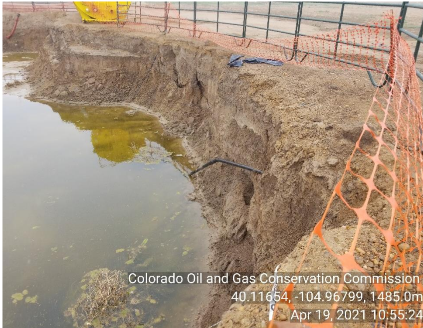
Photo 23 Piping cut and in water
