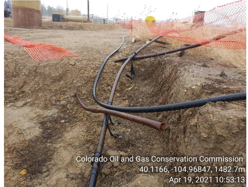
Photo 14 exposed lines not plugged or capped.
