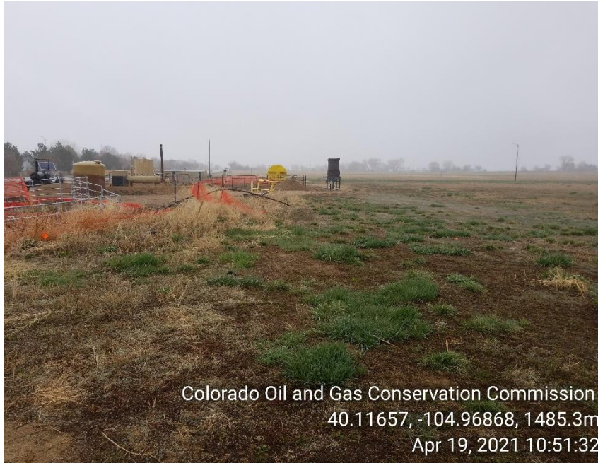
Photo 9 No BMP's around work site to protect run on or run off.
