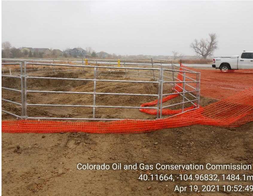
Photo 13 Improper safety fence around work site.
