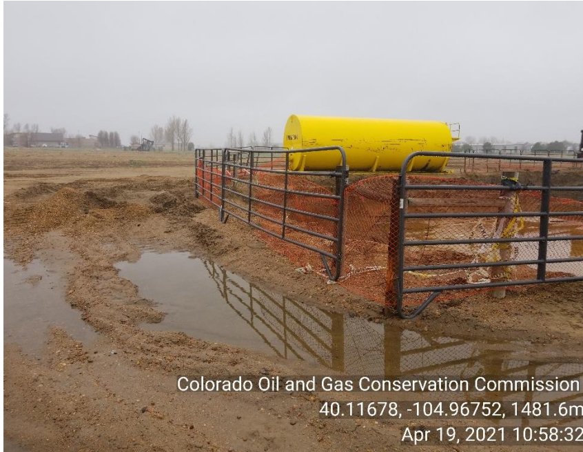
Photo 36 Improper fencing around open excavation and work site
