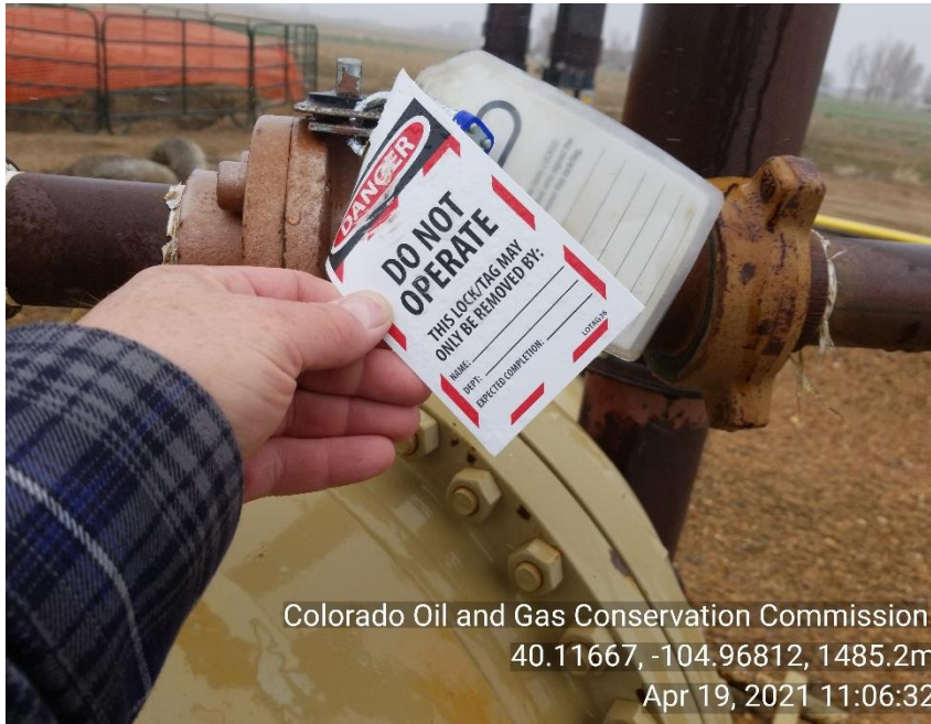
Photo 45 Separator not properly LOTO
