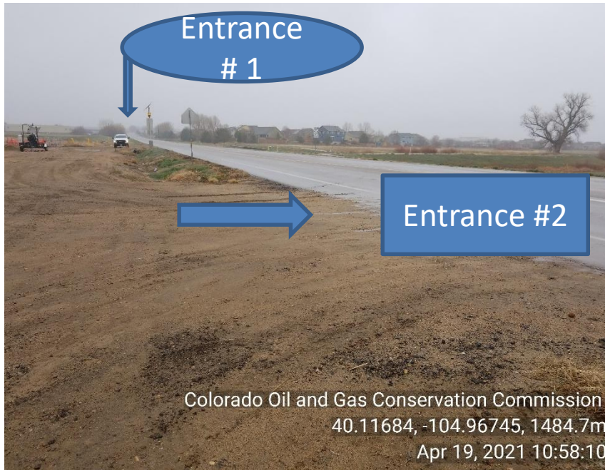
Photo 34 not tracking pad BMP
