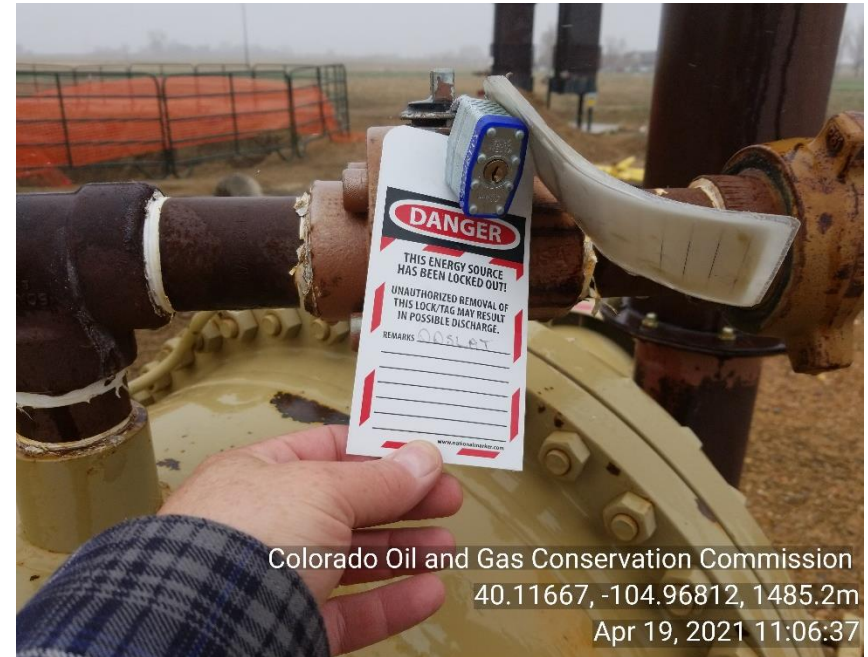
Photo 46 Separator not properly LOTO.
