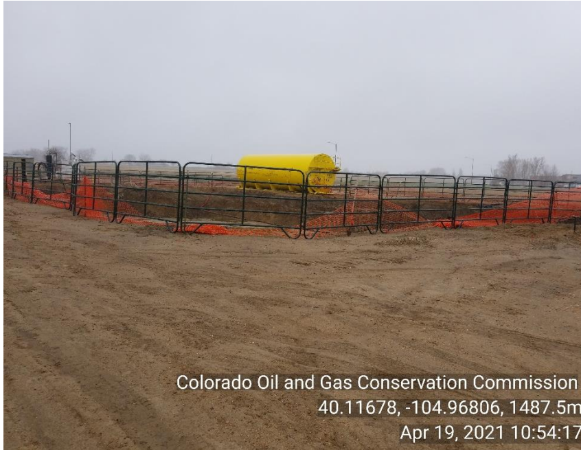
Photo 19 improper fencing around open excavation and work site.
