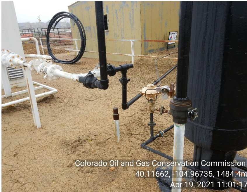
Photo 40 Valves to sales meter in the open position
