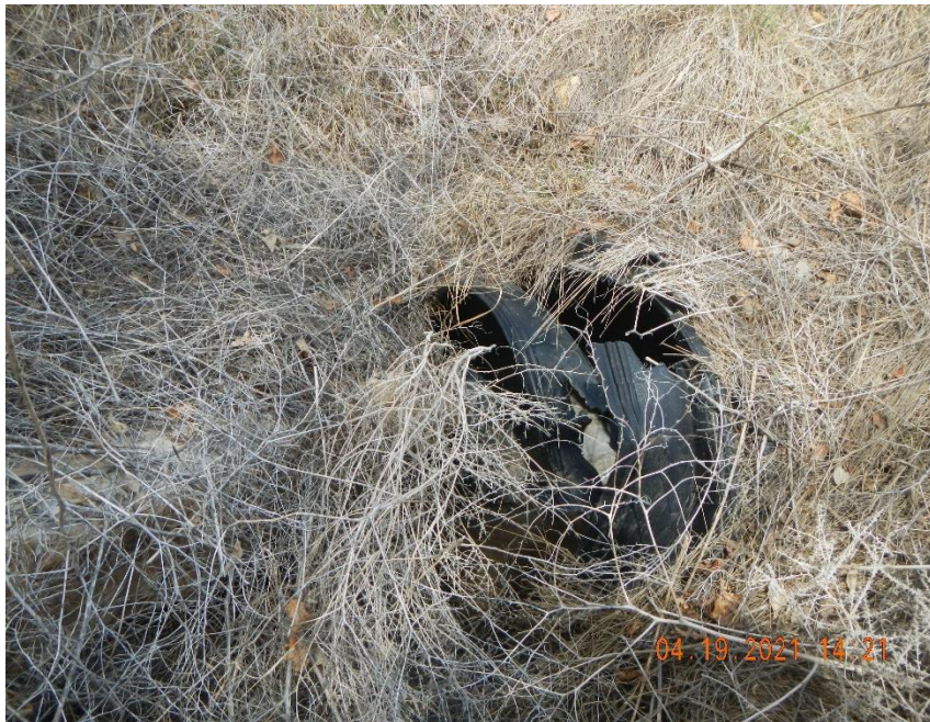
Damaged culvert.
