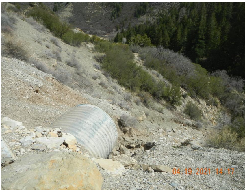
Erosion created from flow of culvert.
