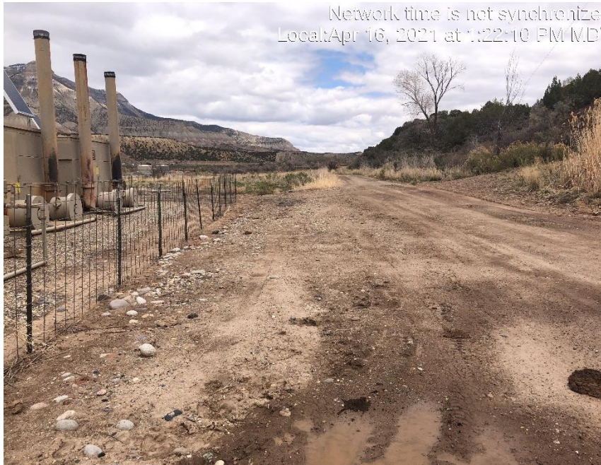
Photo #3522 no form of tracking control at entrance to location.
