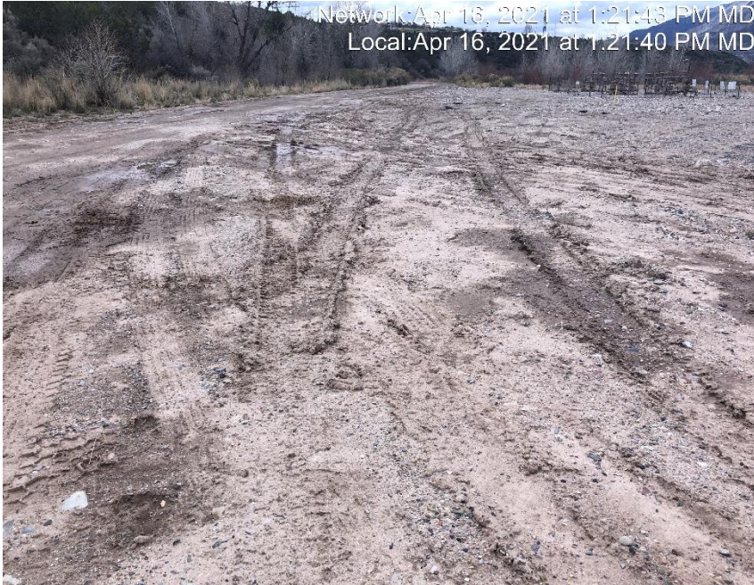
Photo #3520 Location lacks stabilization
