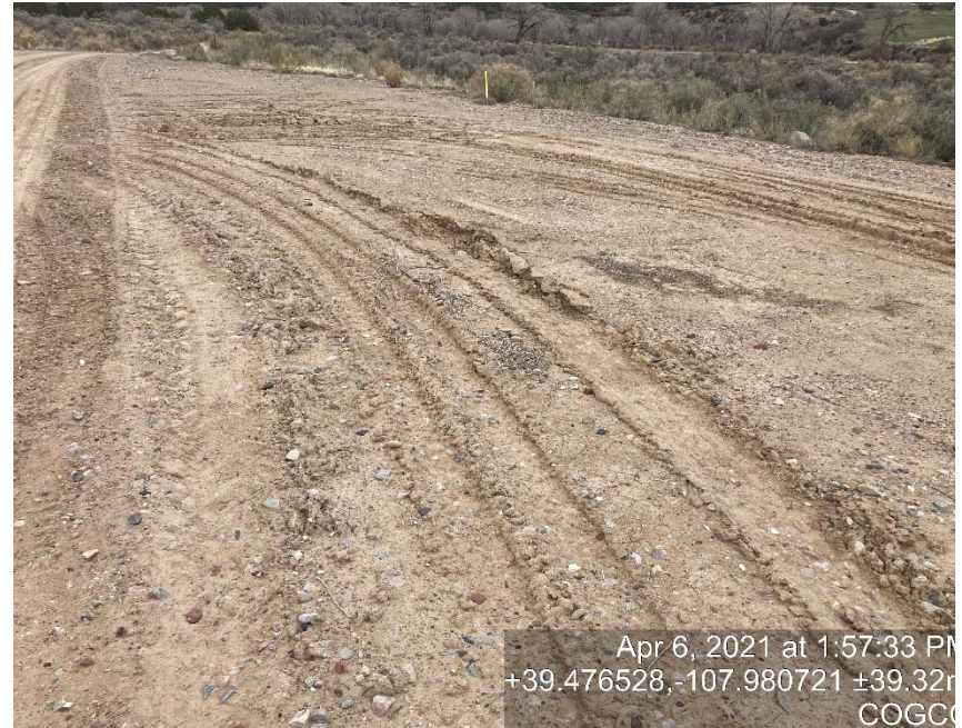
Lack of stabilization/compaction
