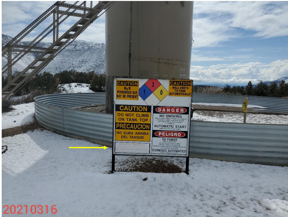
Photo 6: Photo of signage at the tank. Photo shows the emergency contact label on the sign is fading, and becoming difficult to read. Maintenance advised. .
