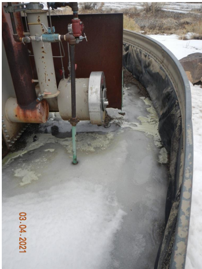
Photo#4: Possible Tank leak.
