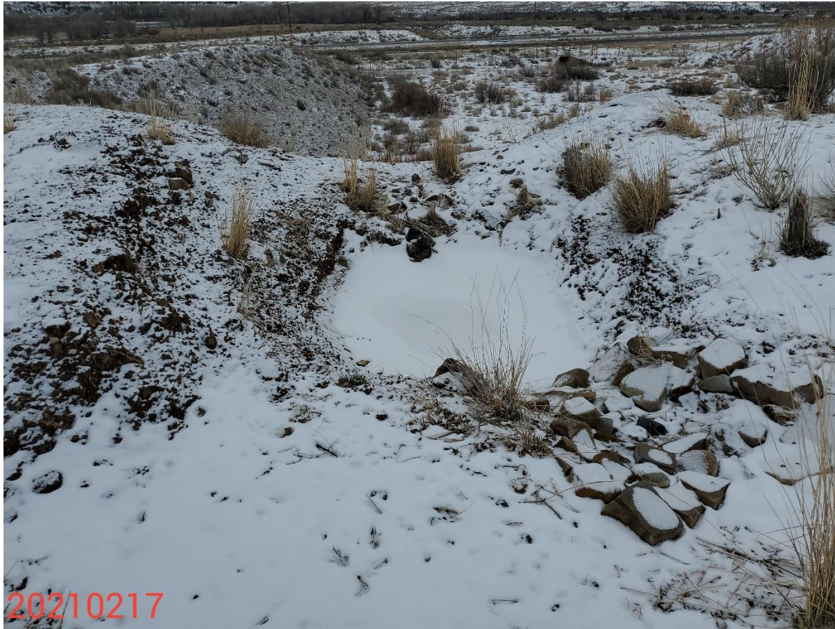
Photo 10: Photo shows the western-most sediment trap on the south end of the Location. BMP has been constructed with a slope-drain.
