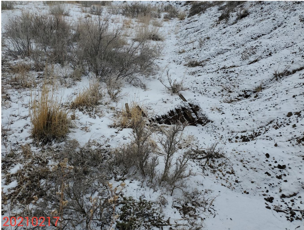
Photo 12: Photo taken from west of the drain outlet (photo 11), facing west. Photo shows hay bale control measure; BMPs has not been maintained in proper functioning condition.
