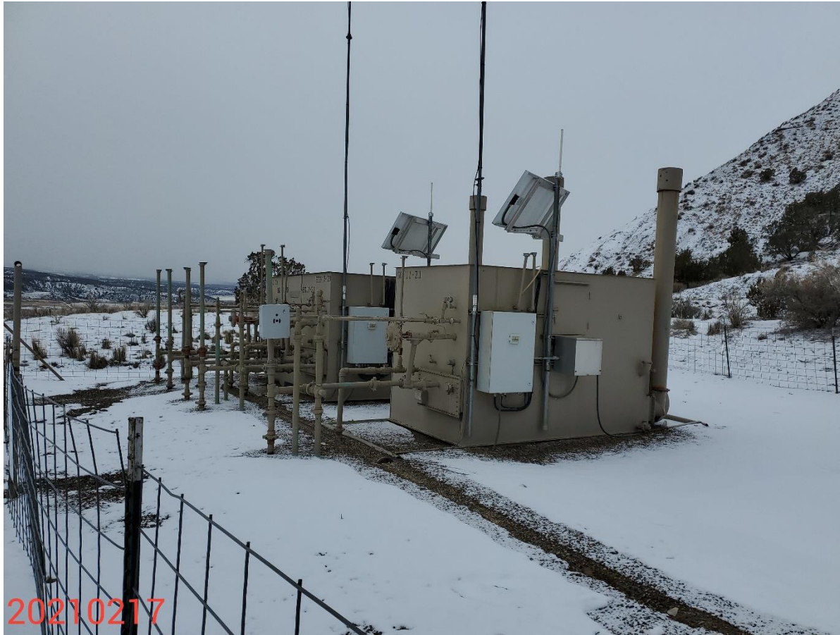
Photo 6: Photo shows separator equipment on the north end of the Location.
