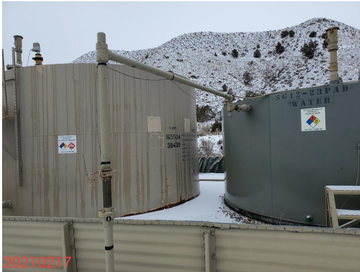
Photo 5: Photo shows 300 bbl “natural gas condensate” and 200 bbl “produced water” tanks and containment bmp on the north end of the Location.
