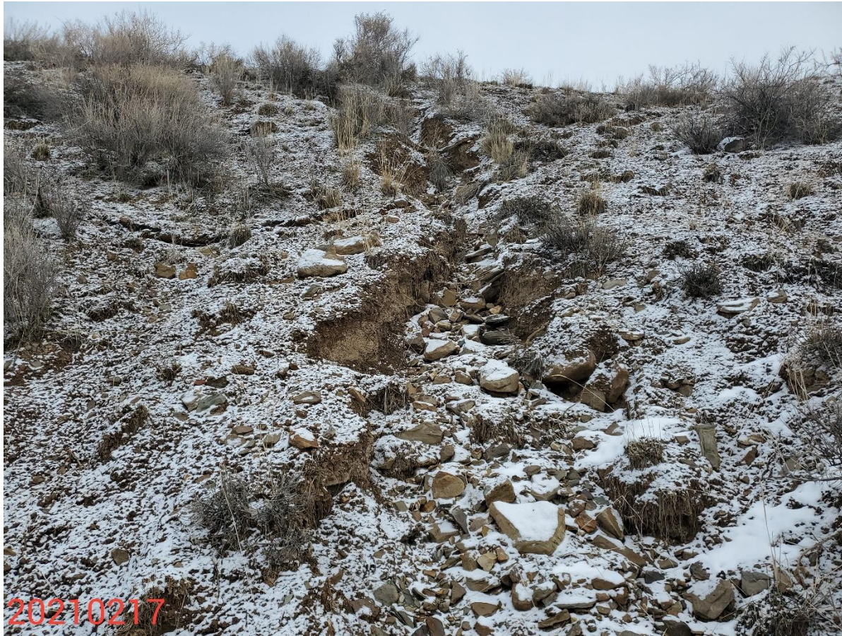
Photo 13: Photo taken from the slopes on the south end of the Location. Photo shows gully erosion. BMPs missing or insufficient to stabilize slopes.
