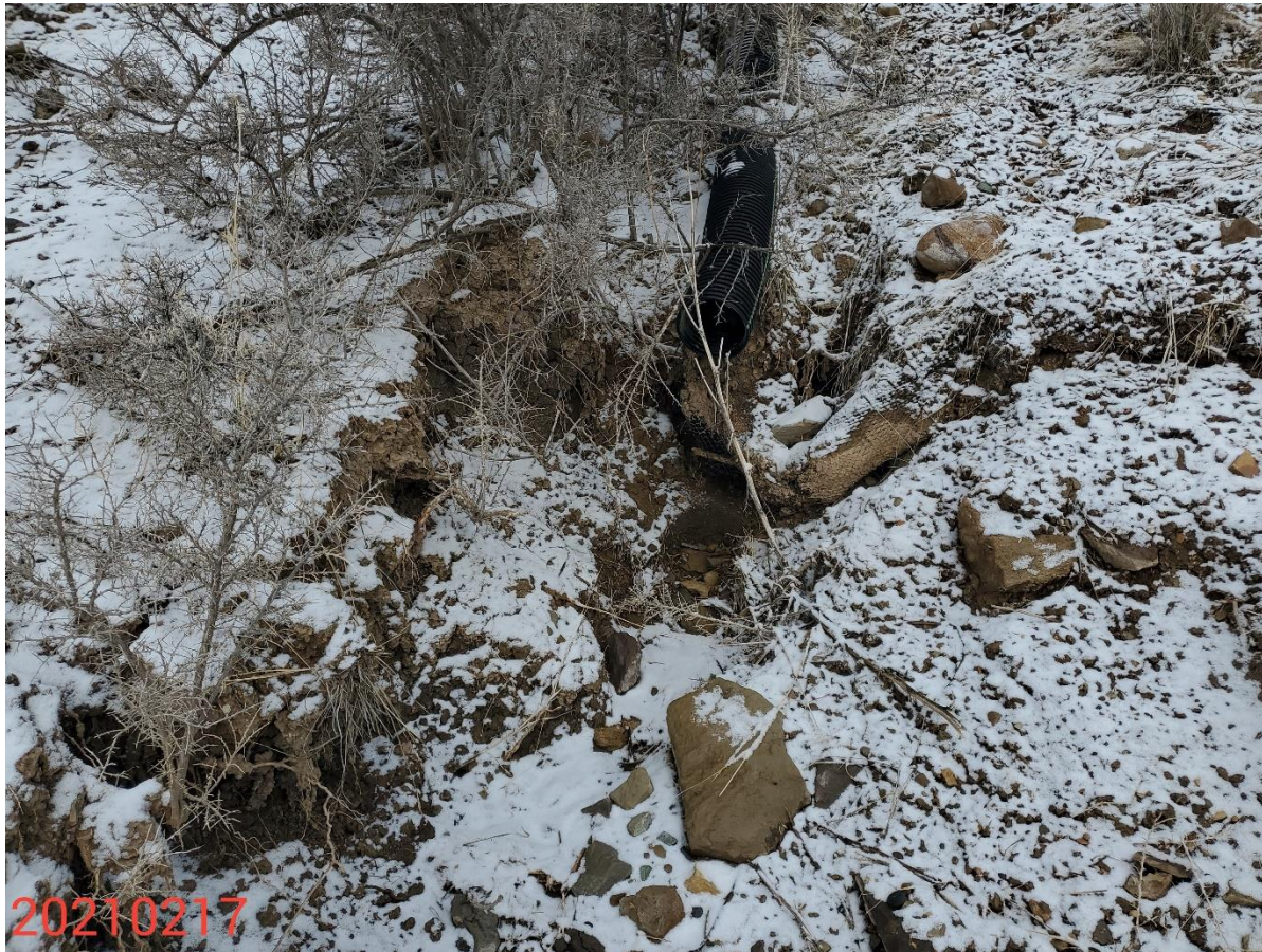
Photo 11: Continued from photo 11. Photo shows outlet of slope drain. Photo shows outlet has not been constructed in accordance with good engineering practice; erosion degradation evident.
