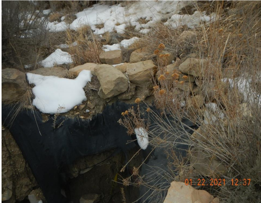
Erosion damage from culvert outlet.
