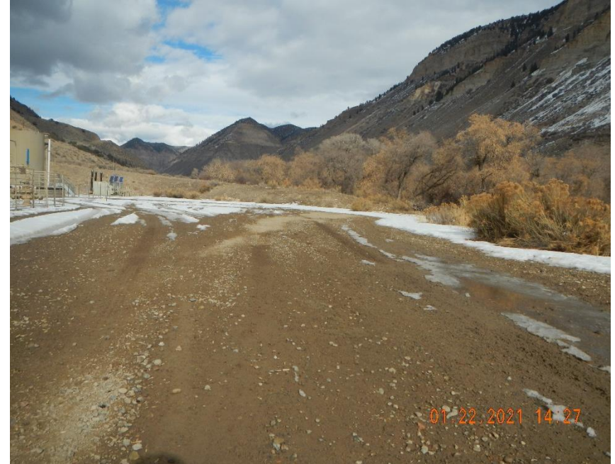
Location shows signs of lack of stabilization BMPs
