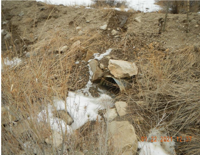
Sediment build up in culvert outlet.
