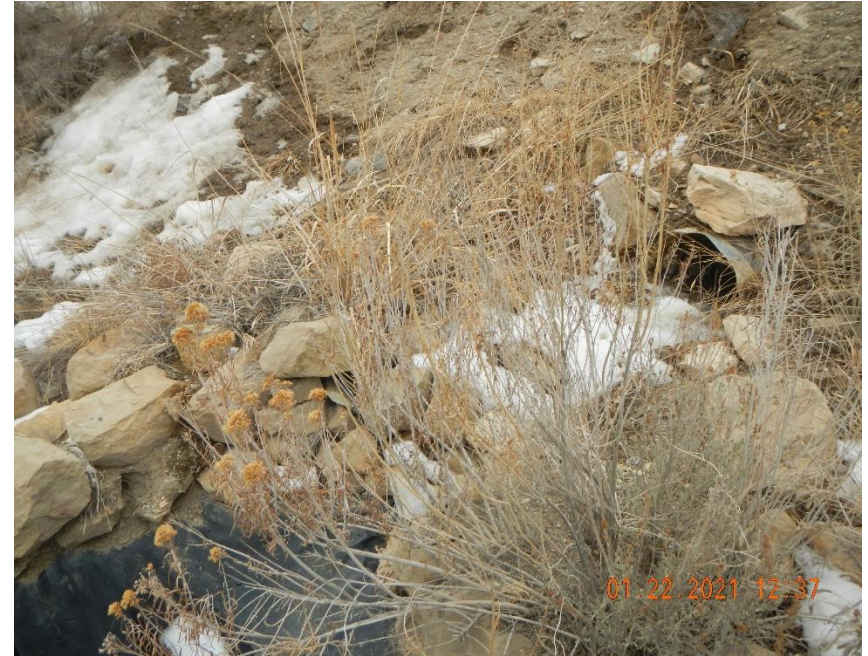
Erosion damage from culvert outlet.
