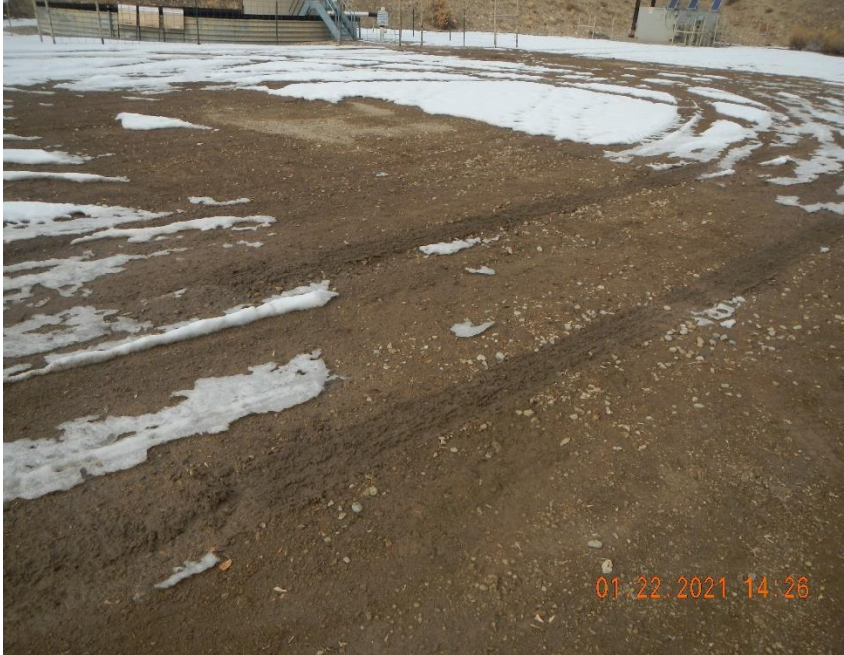
Location shows signs of lack of stabilization BMPs
