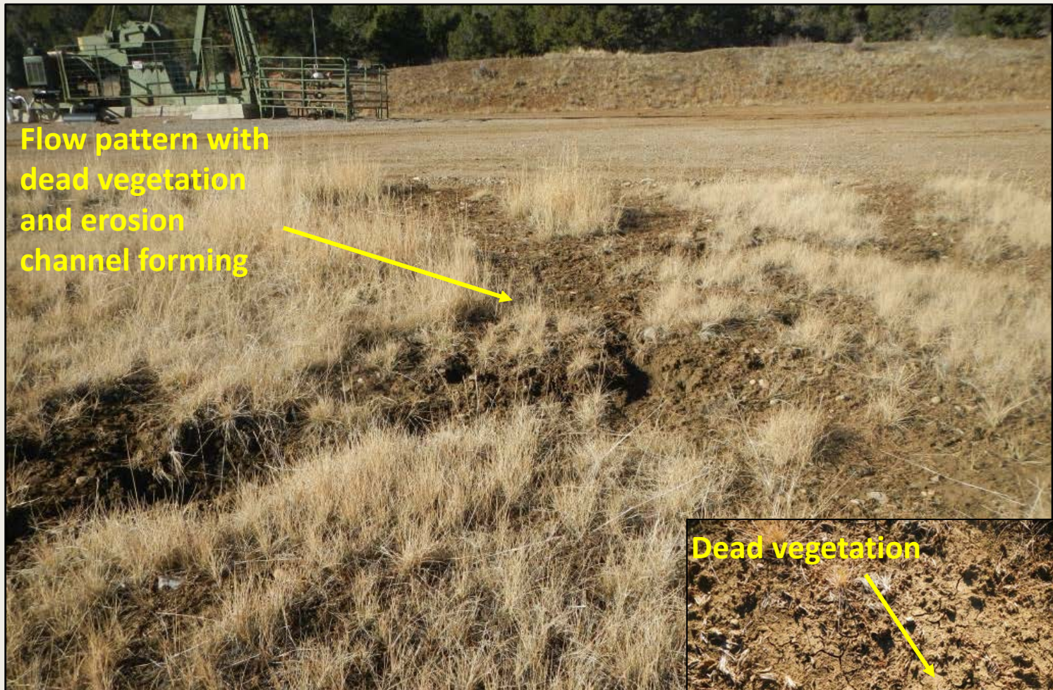
Photo 3. View of area in the eastern project area where stormwater pattern from the well pad is resulting in vegetation die-off and erosion. Channel is approx. 10 inches wide and deep. Inset in right hand corner shows vegetation killed in flow pattern.
