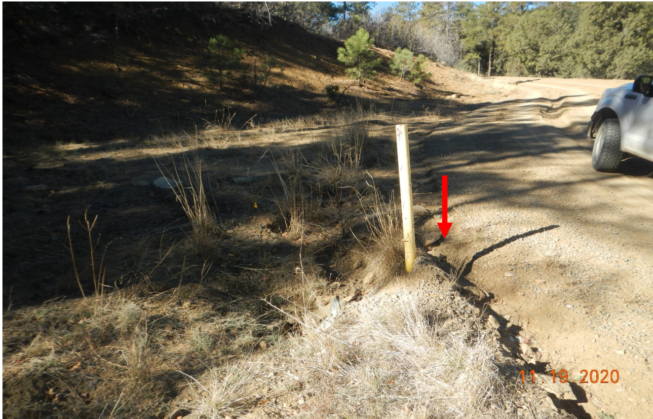
Photo 1. Stormwater is not being diverted toward the culvert which is causing erosion further down the road. Culverts need to be maintained for stormwater diversion.
