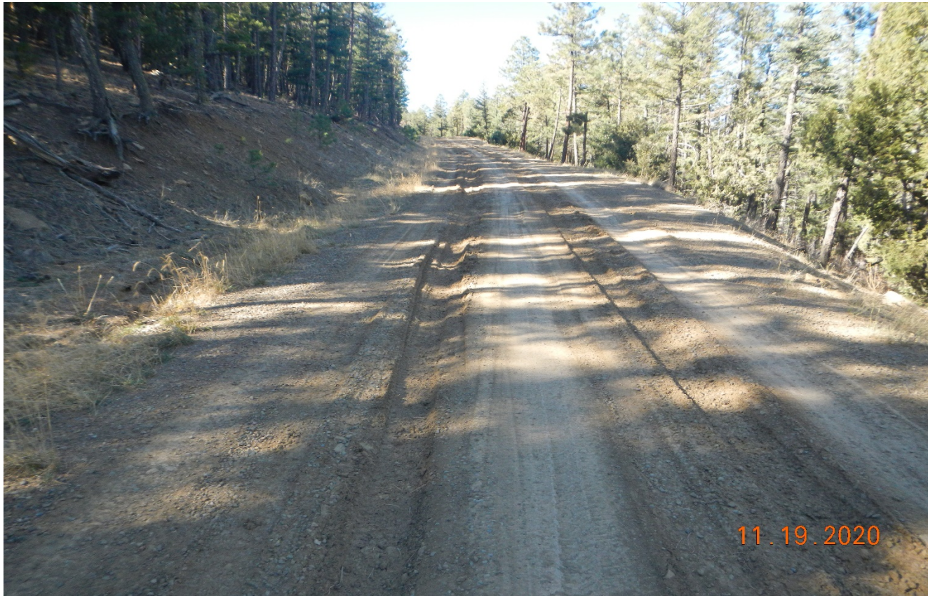
Photo 2. There is vehicle rutting occurring along the road which will only worsen if not repaired. The roads need to be maintained.
