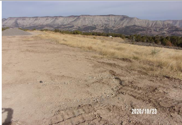
Erosion Channels on the HDU 21-41-H Pad
