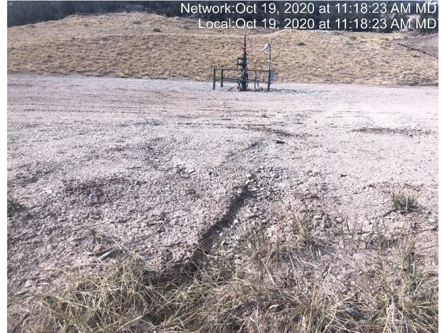
Photo #2043 Channel erosion accruing on east side of location.
