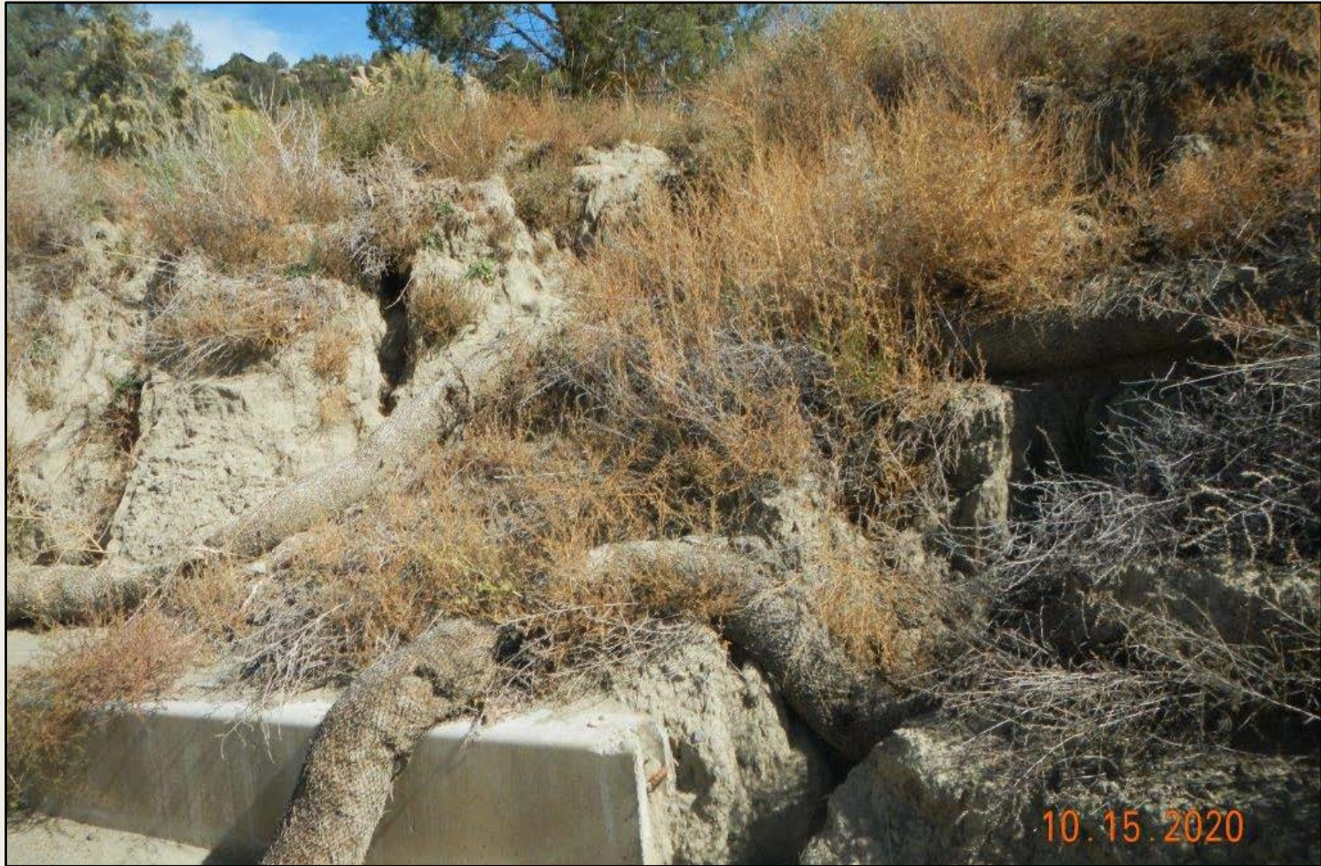
Photo 2. View of erosional channels and failed wattles within the southeastern project area. Erosional channels up to approximately 4 feet deep present here.
