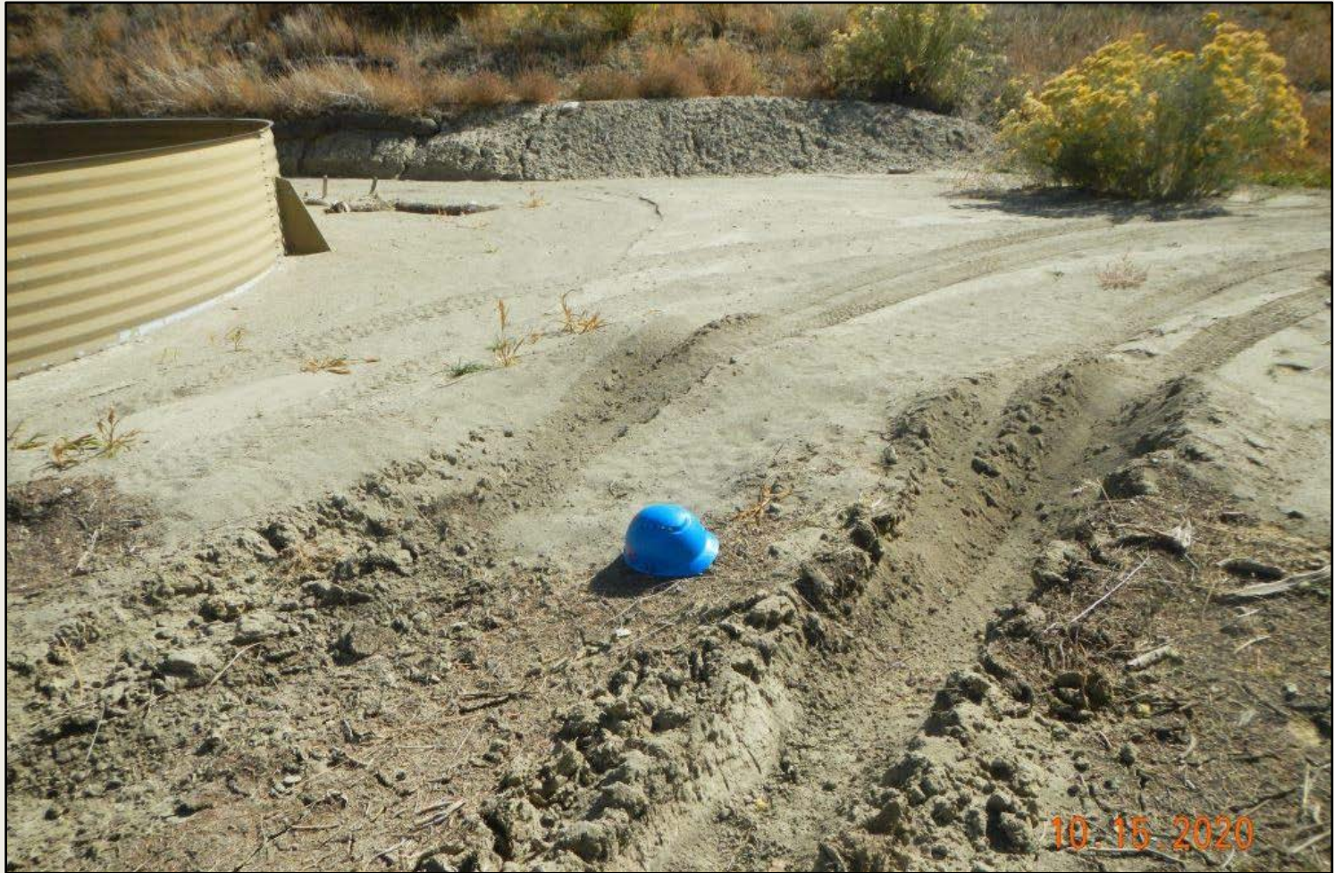
Photo 4. View of sediment deposition, up to 2.5 feet deep within the southern project area.
