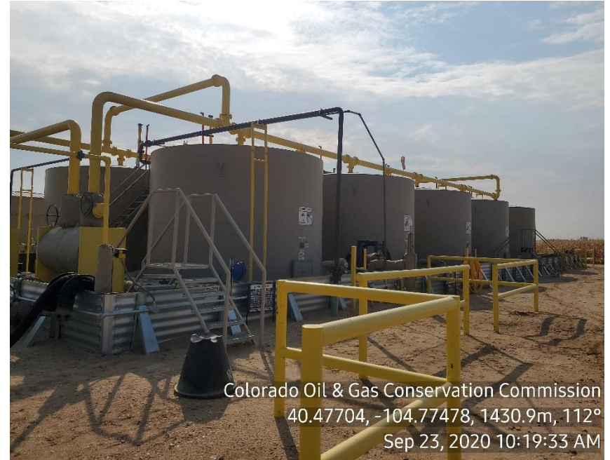
Photo 2: Tank Battery
