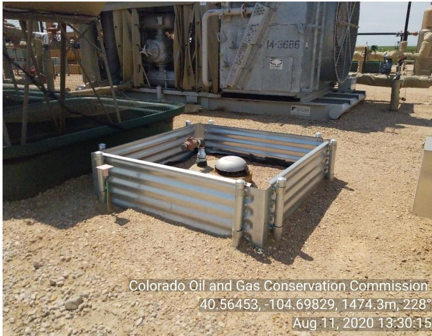
Photo 7: No labeling on tank
