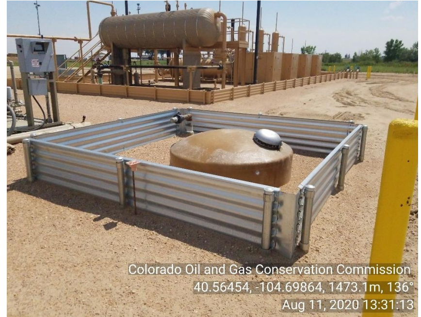
Photo 6: No labeling on tank
