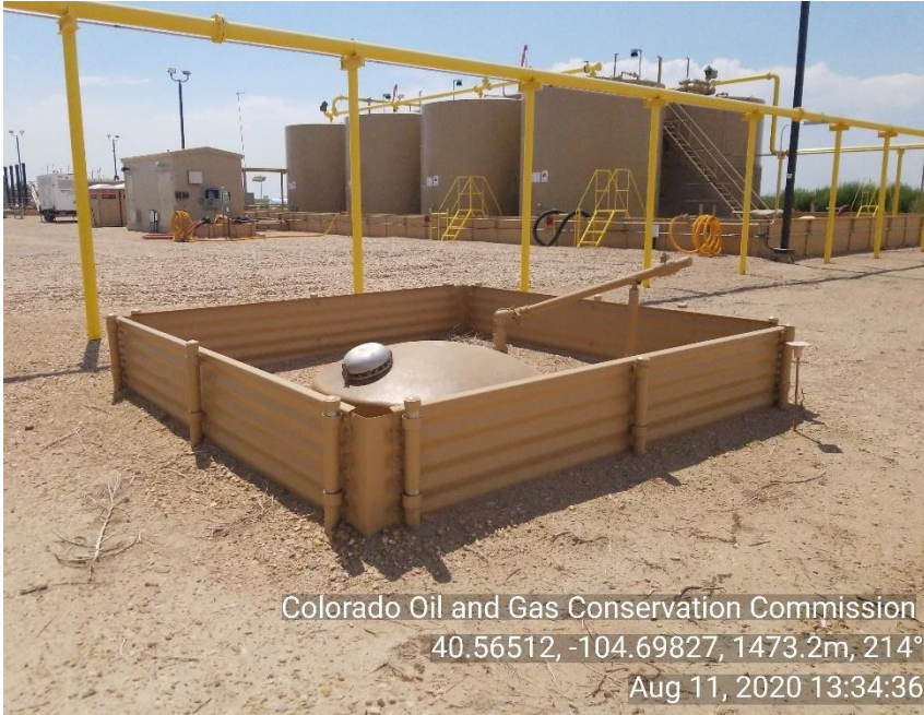
Photo 5: No labeling on tank
