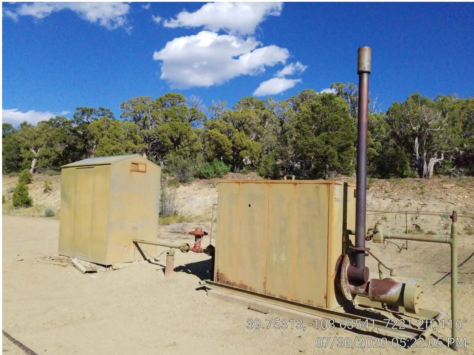
Photo 4. Meter building & separator.
