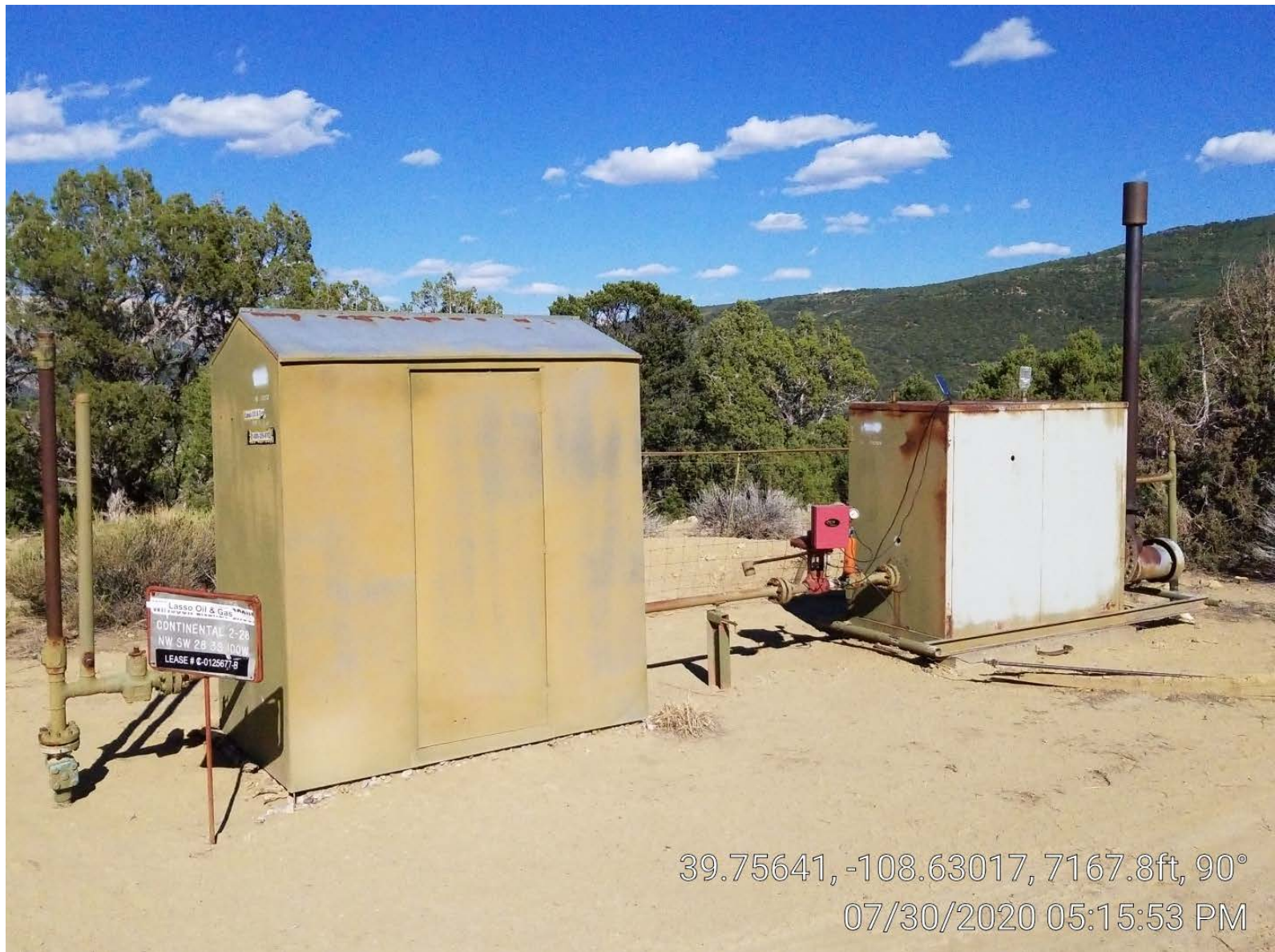
Photo 3. Meter building, pit, separator.
