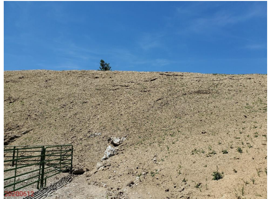
Photo 4: Photo taken from the southwest end of the Pad. Photo shows Operator has used a hydromulch to stabilize the seeded soils of the Location. Photo shows areas of the cut slope where soils show sign of destabilization.
