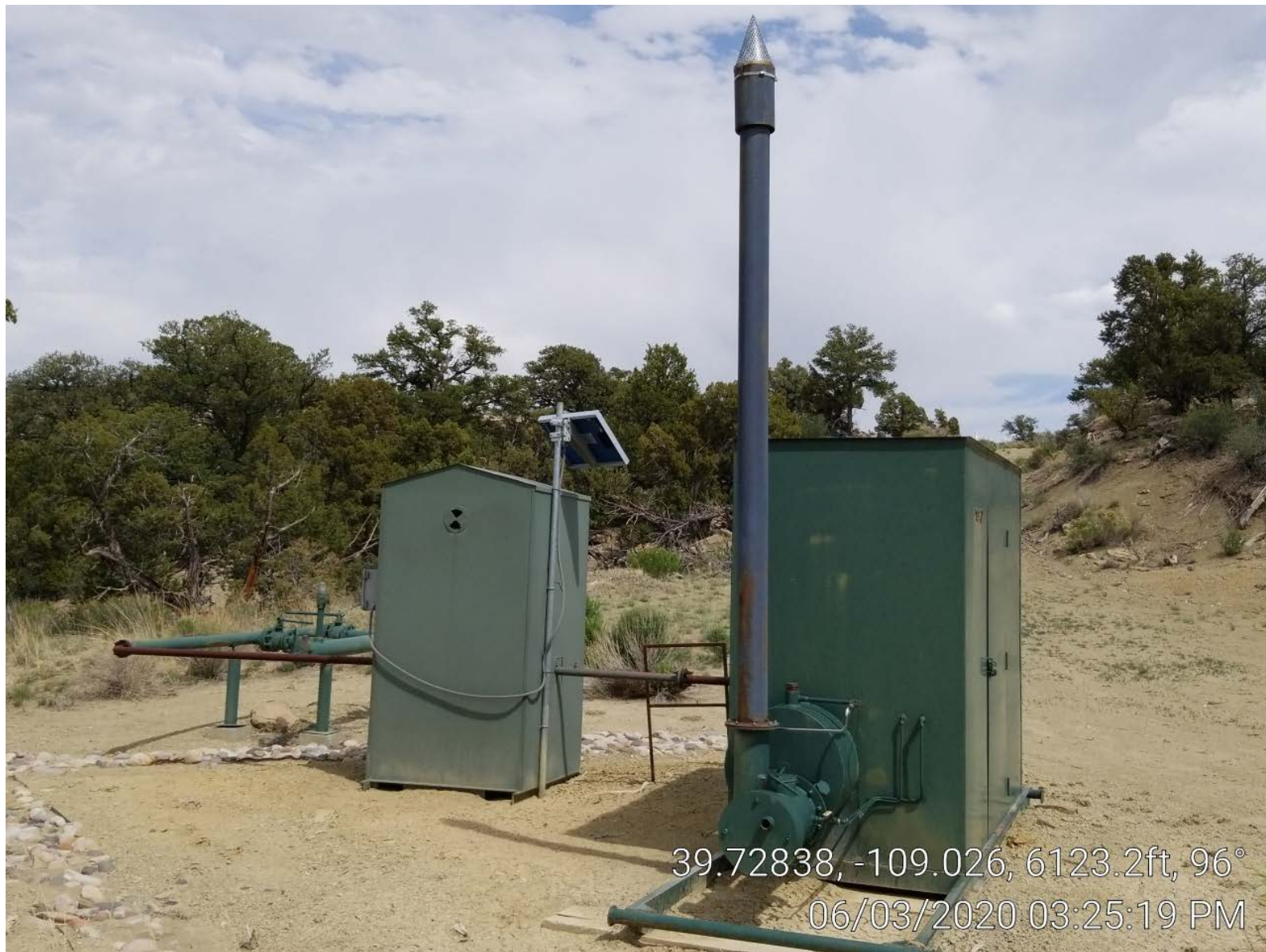
Photo 3. Meter building & separator.
