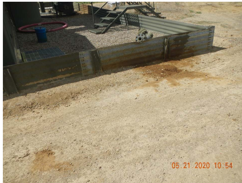
Photo 2. Stained soil at tank battery.
