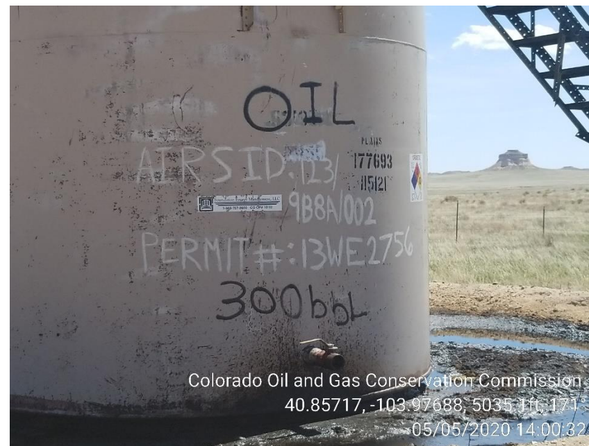
Photo 2 – Crude Oil tank with free standing fluid
