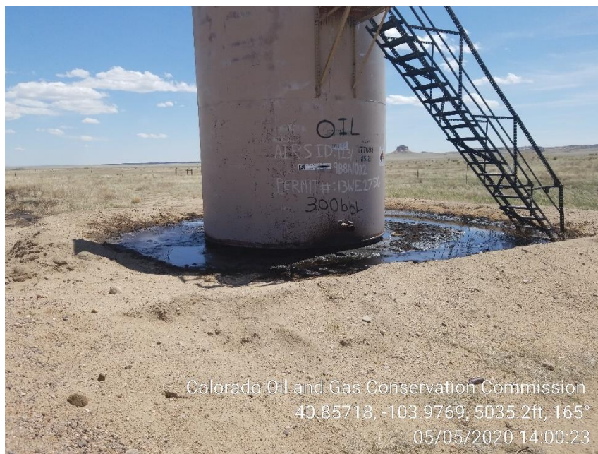
Photo 1 – Crude Oil tank with free standing fluid
