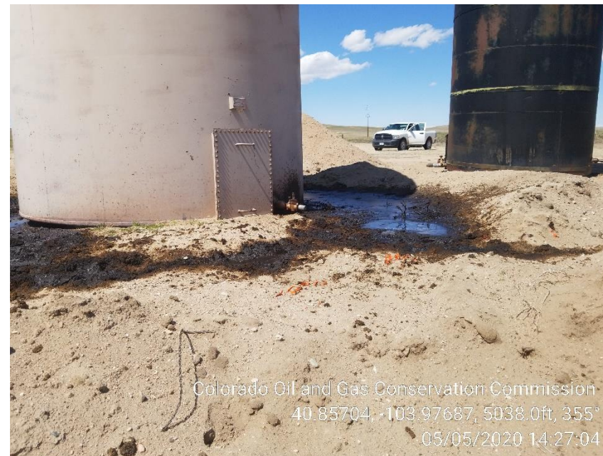
Photo 6 – Back of Tank and compromised containment
