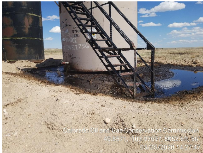
Photo 7 – Crude Oil tank with free standing fluid
