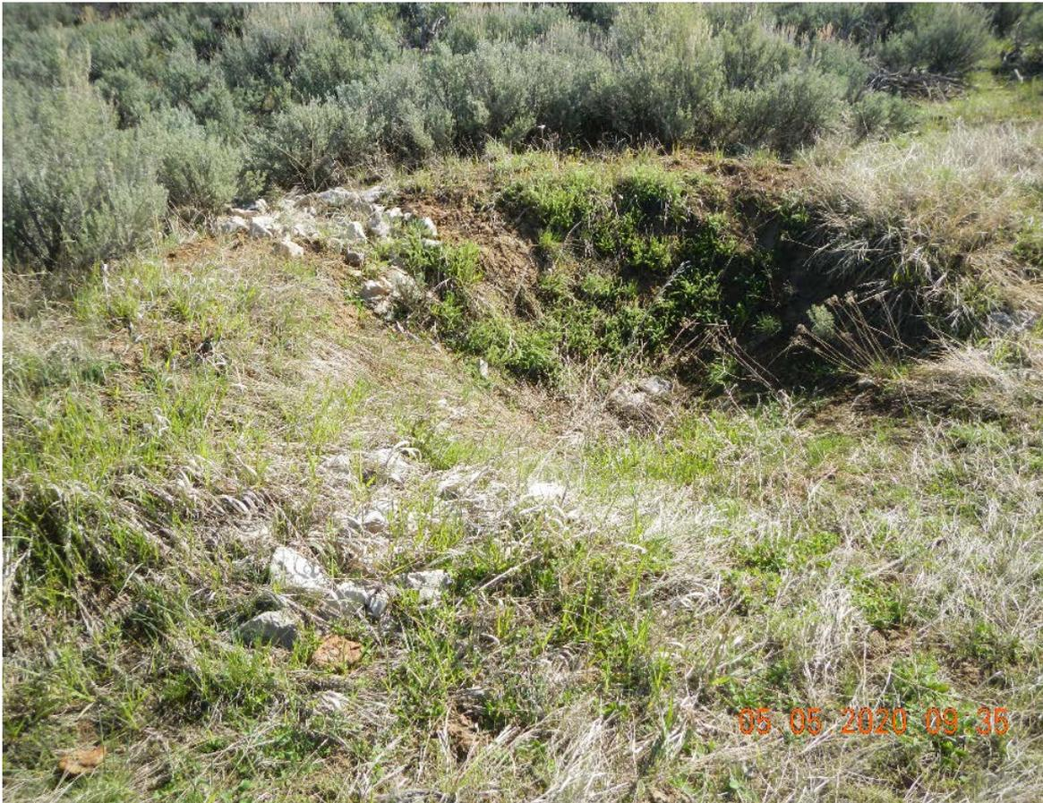
Photo #14 Second Stormwater Infiltration Pond #2. Note rip-rap.
