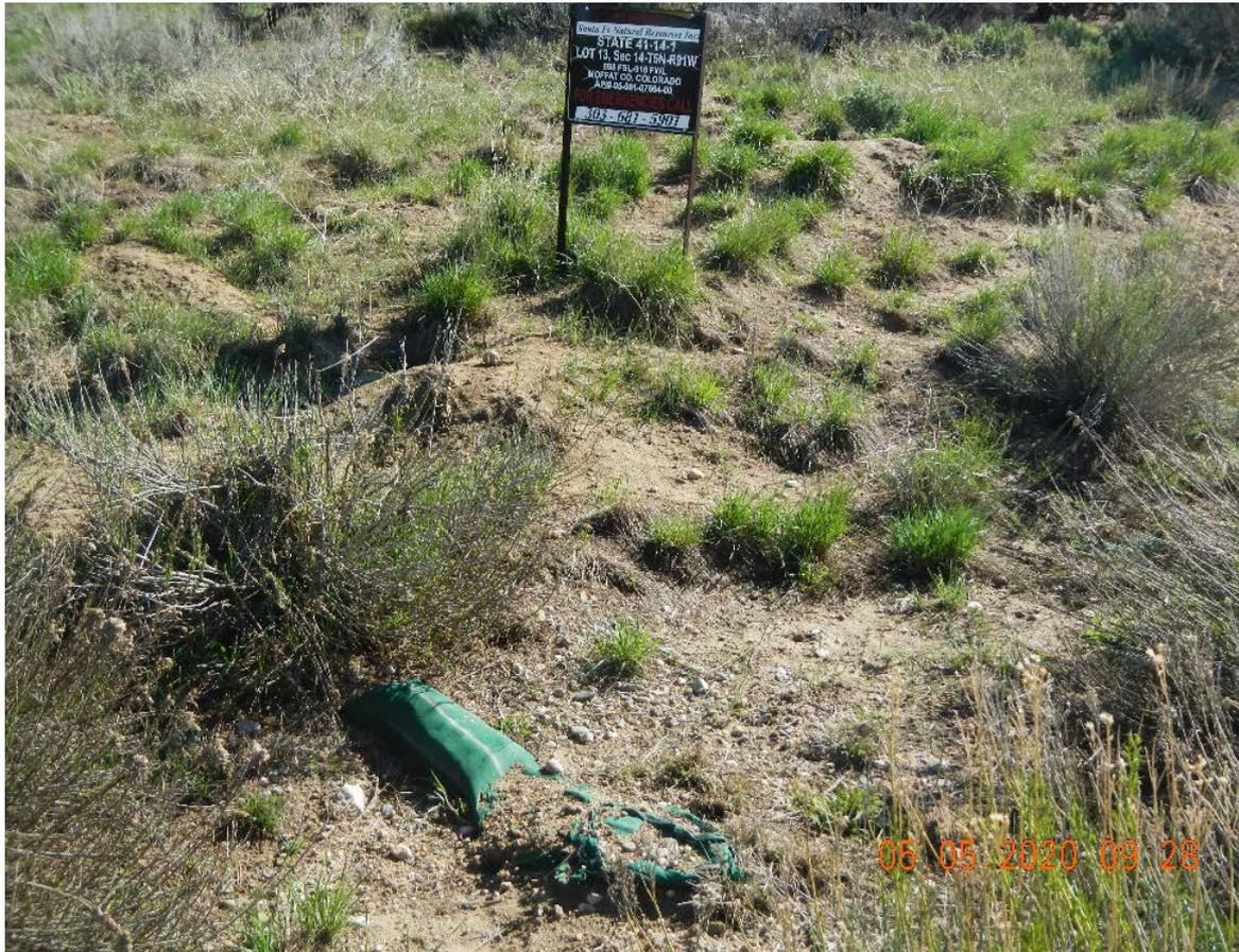
Photo #2 stormwater BMP's witness around pad; sandbags, ditches, 3 small (10 diameter) infiltration ponds
