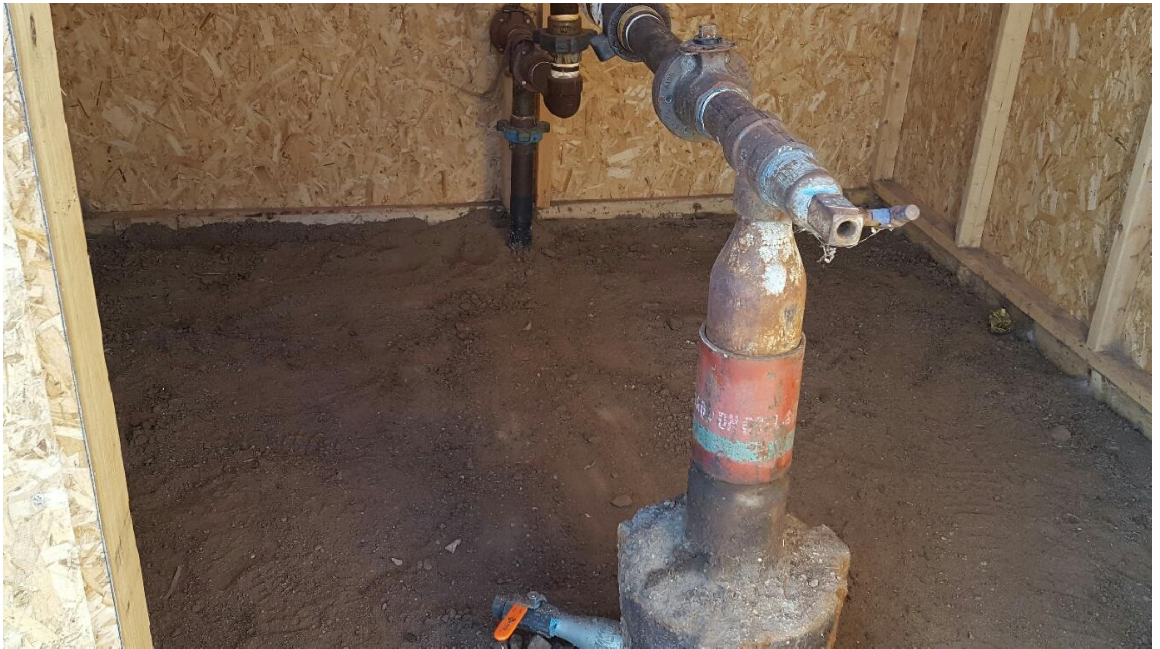
Figure #1 Unused riser has been removed
