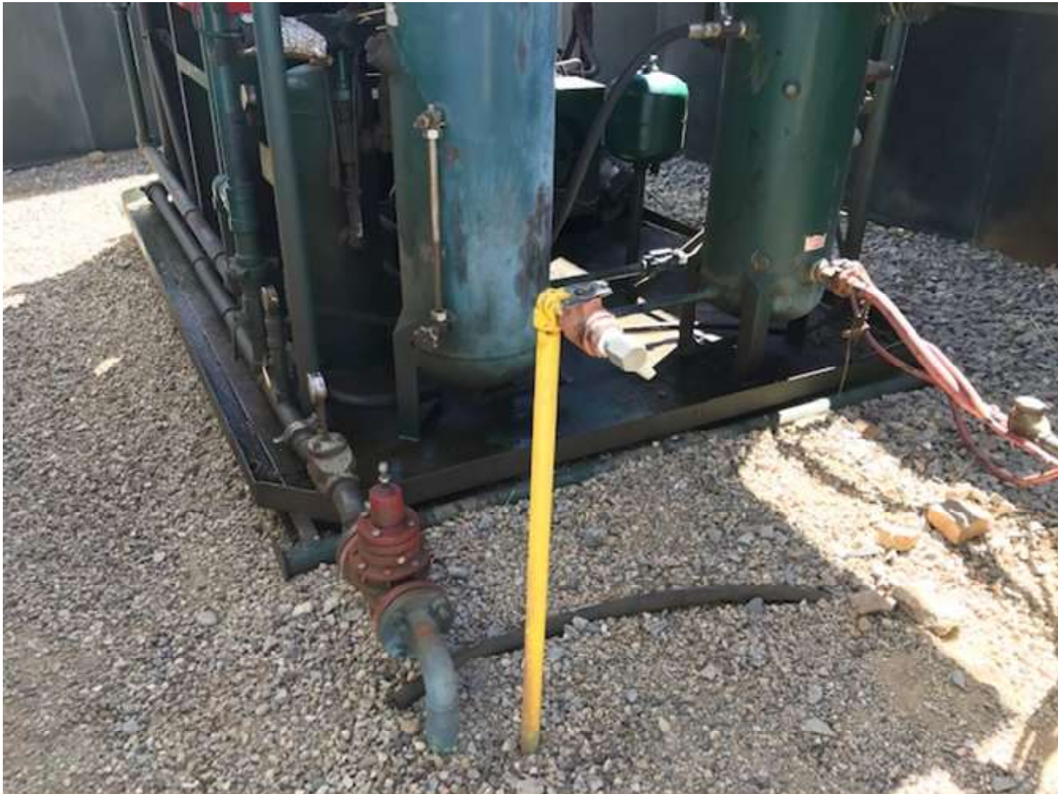
PHOTO 5: THE FLUID ACCUMULATION WAS REMOVED FROM THE LIQUID RING ENGINE SKID.
