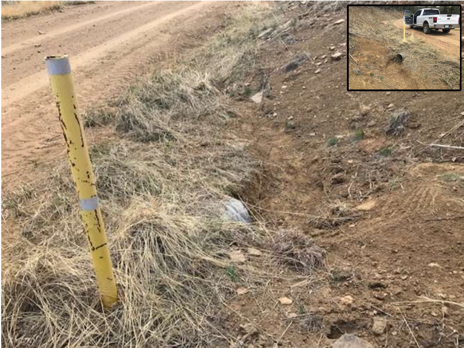
PHOTO 2: THE SEDIMENT ACCUMULATION WAS REMOVED FROM THE CULVERT INLET ALONG THE MAIN LEASE ROAD.
