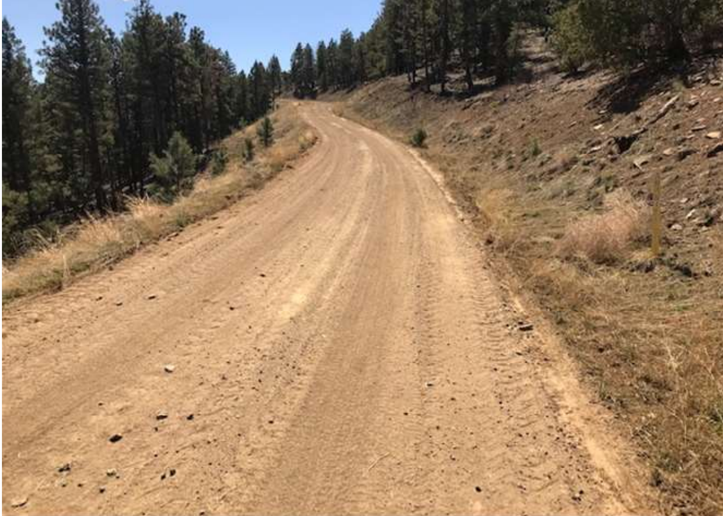
PHOTO 1: THE MAIN LEASE ROAD WAS SURFACE CROWNED TO ESTABLISH SHEET FLOW AND ELIMINATE THE TIRE RUTS.
