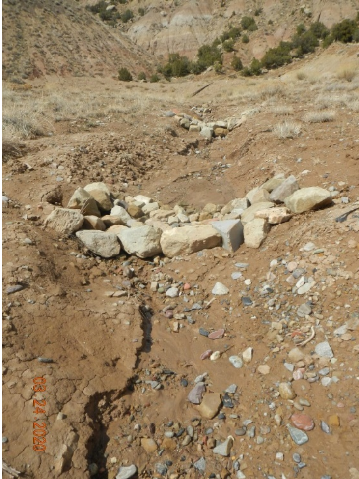
Photo#6: BMPs along East side of site.
