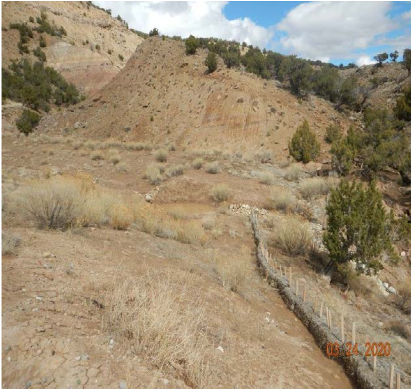
Photo#2: BMPs installed as a series.
